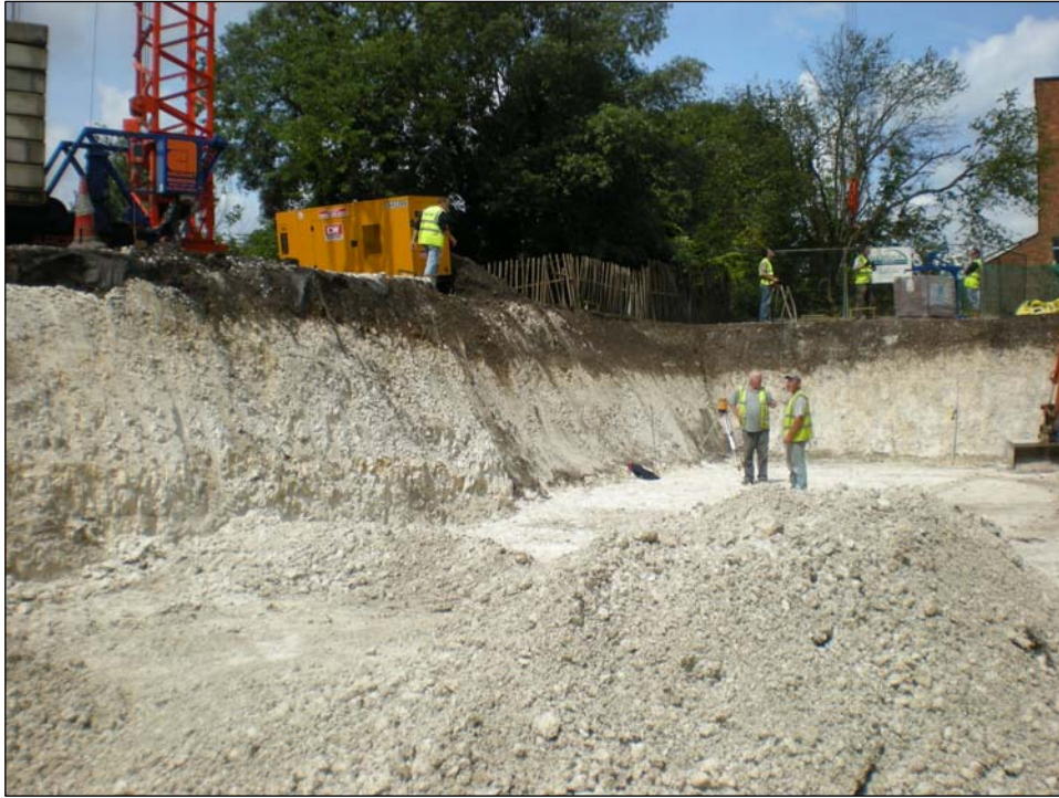
3 View inside the foundation pit. Looking north-west
