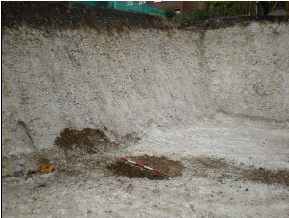
4 Northern corner of foundation pit showing Roman well F2014. Looking north.
