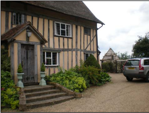
1 General view of the site. The outbuildings under renovation are in the background.
