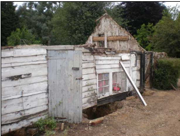
3 Outbuildings under renovation. Looking north.
