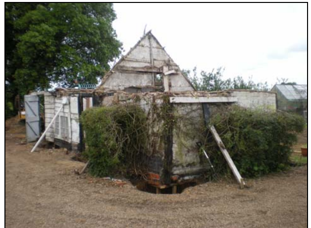
4 Outbuildings under renovation. Looking south-west.
