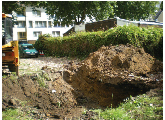
DP 4. Trial Trench 1 under excavation. View NE.
