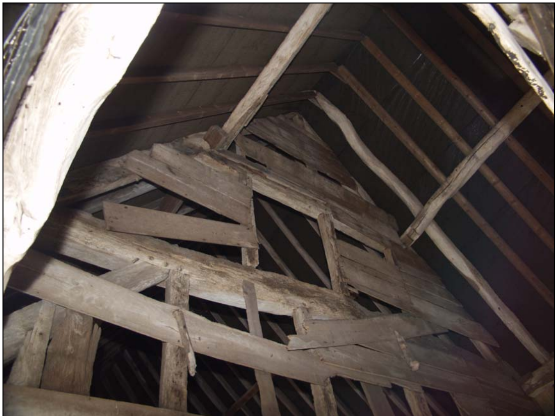
Plate 8 North side of the open-bay of Unit 4 showing the formerly external wall of the 15th century barn, taken from the south-west (26)
