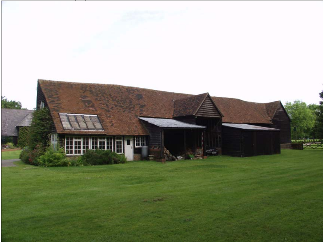
Plate 2 View of the east side of the assessment structure, taken from the south-east (05)
