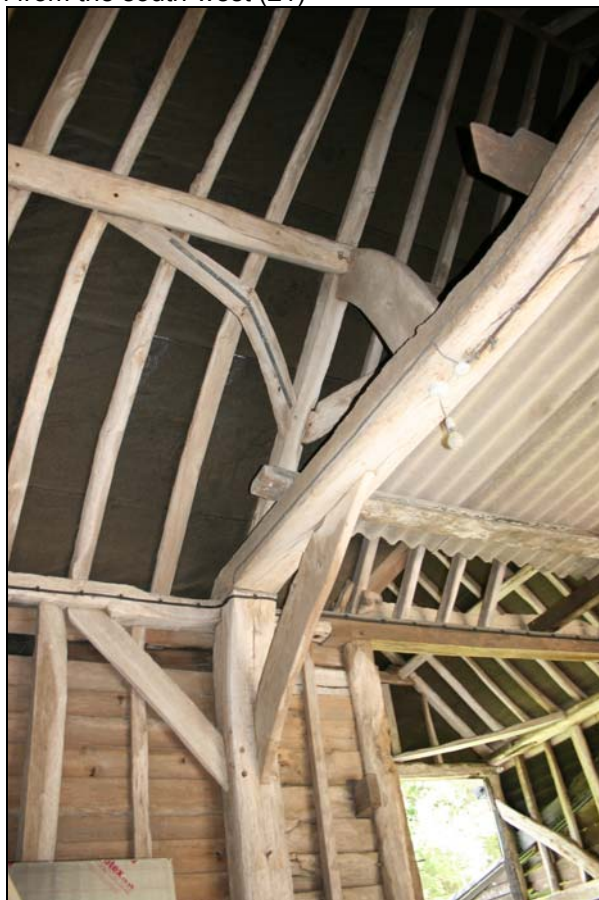
Plate 6 Detail of the inner truss construction of Unit 4, taken from the east (37)
