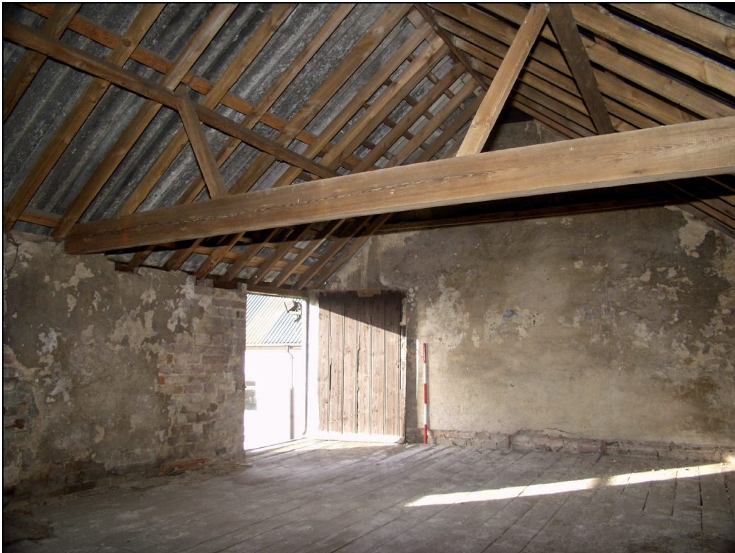
4 Interior of first floor of former stable, taken from the north-east (16)
