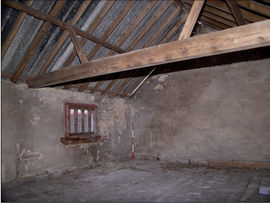
3 Interior of first floor of former stable, taken from the south-west (15)
