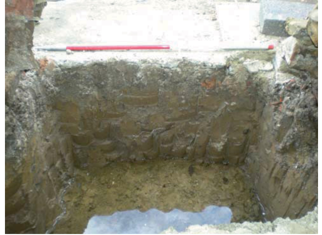
DP 32. Former stable, Building A, NW corner. Foundation pit/trench. Taken from S.
