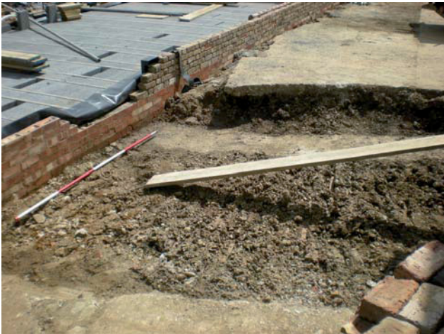
DP 37. Foundations for the link building. Taken from SW.
