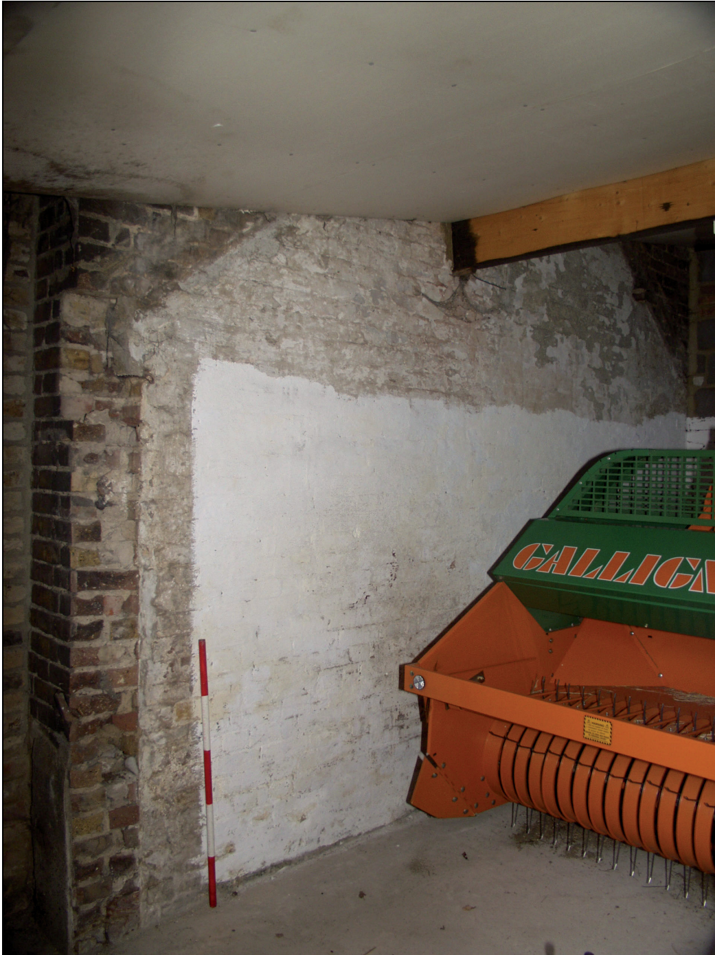
5 East end wall of former stable, taken from the south-east (12)
