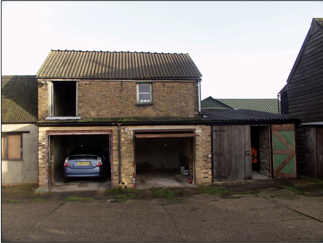
1 Southern elevation of former stable, taken from the south (11)
