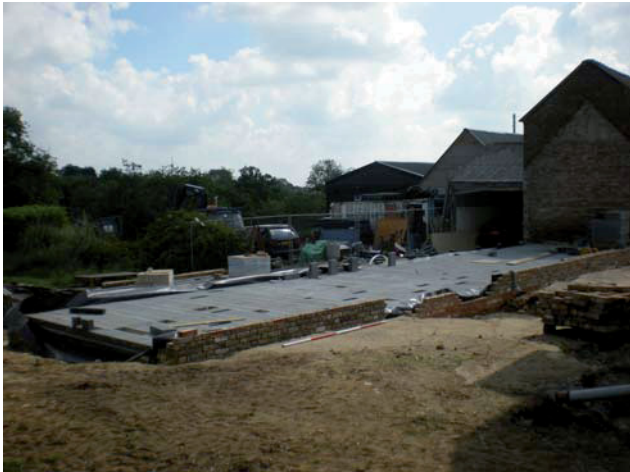
DP 27. Building A. Taken from WSW.
