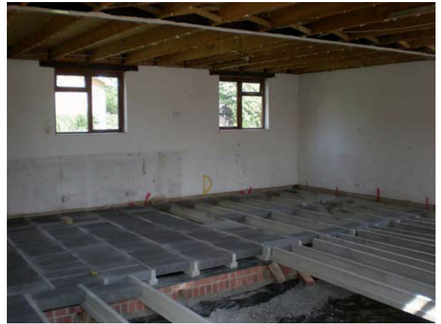
DP 40. Interior of Building B. Taken from SSE.
