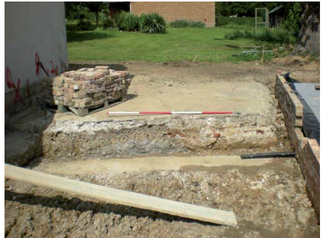
DP 38. Foundations for link building. Taken from E.
