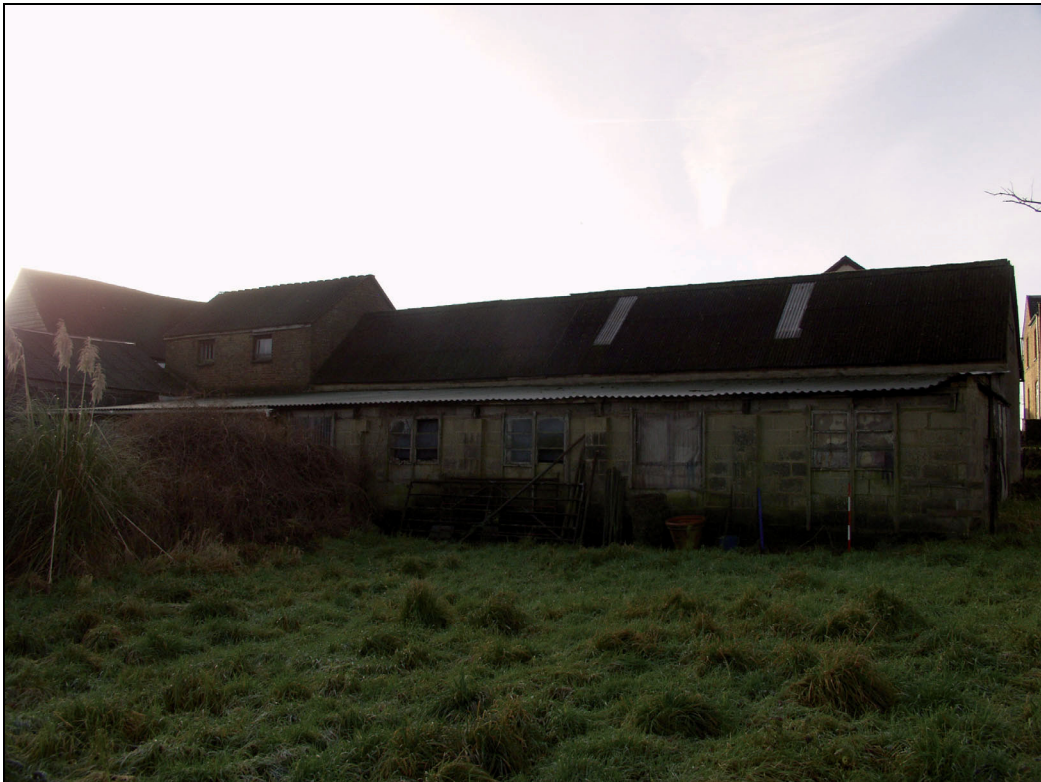
2 Northern elevation of Building A, taken from the north (6)
