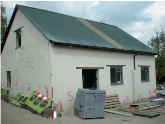
DP 39. Building B. Taken from SSE.
