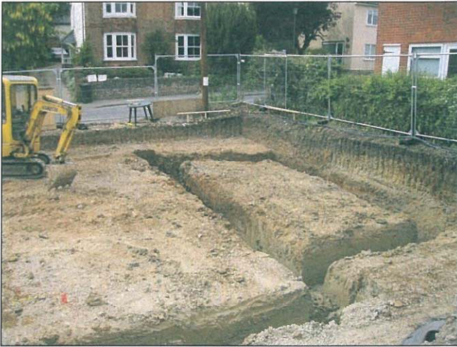
DP 13. Foundation trenches in Plot A, May 2009. Looking north-west.
