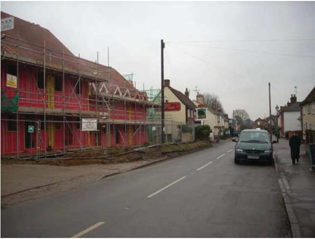
DP 1. High Street, Walkern. Looking from NW. January 2009.
