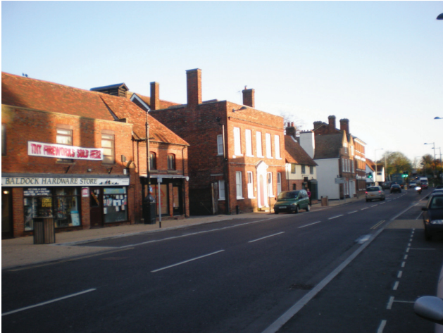
DP 1. Whitehorse Lane, Baldock, Hertfordshire. View N.
