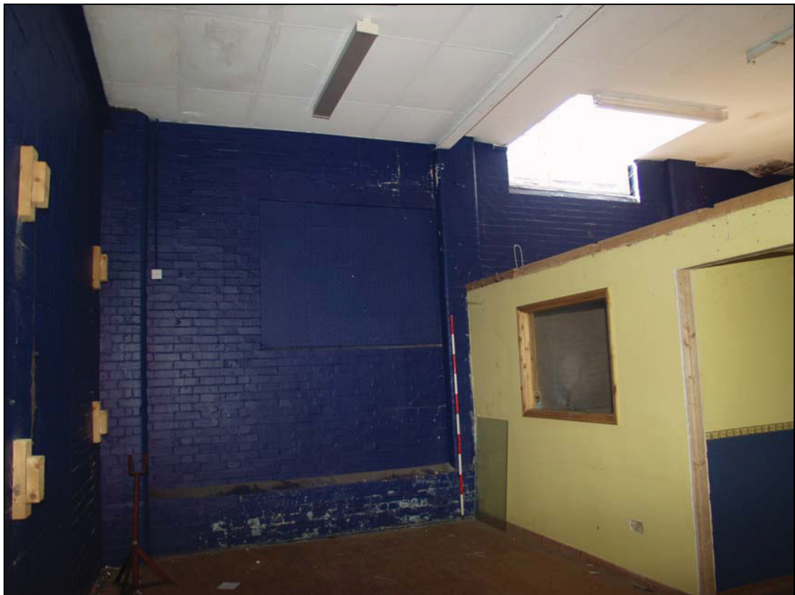
Plate 2 West wall of Unit 2 in Building 1, taken from the east (DP 16)
