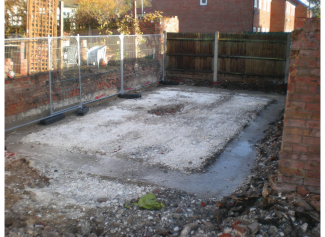
DP 8. N corner of the site. View N.
