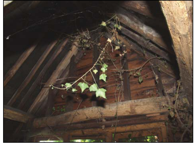
West gable end of Building 3 showing original collar, taken from the north-east
