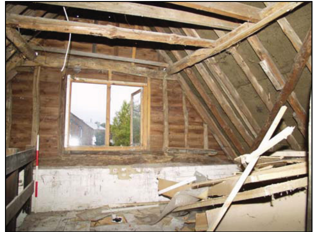
West gable end of Building 3 showing original collar, taken from the north-east
