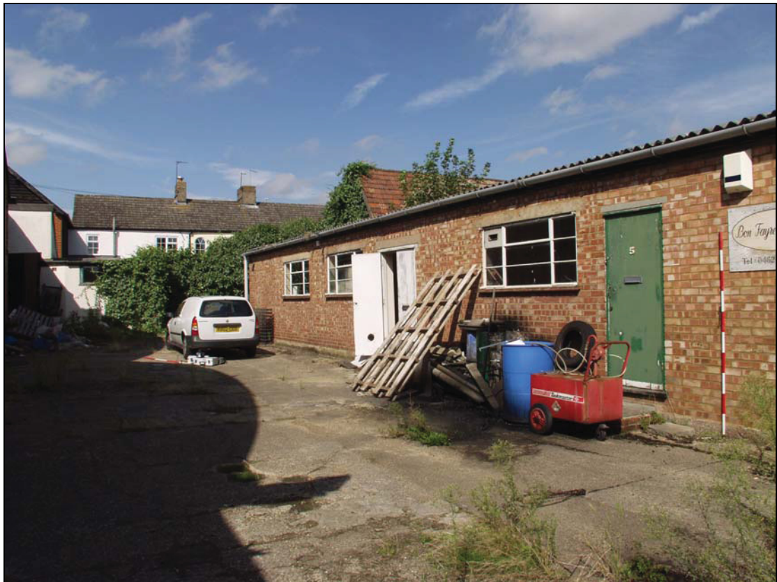
Plate 4 West elevation of Building 2, taken from the south-west (DP 08)
