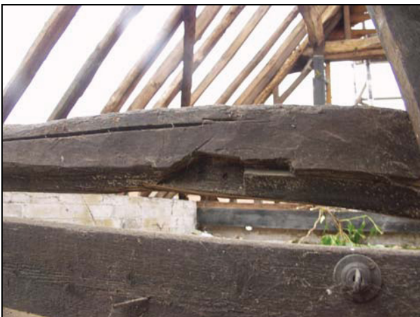
Detail of redundant mortise for a lower brace on the tie-beam of the west truss, Building 3, taken from east
