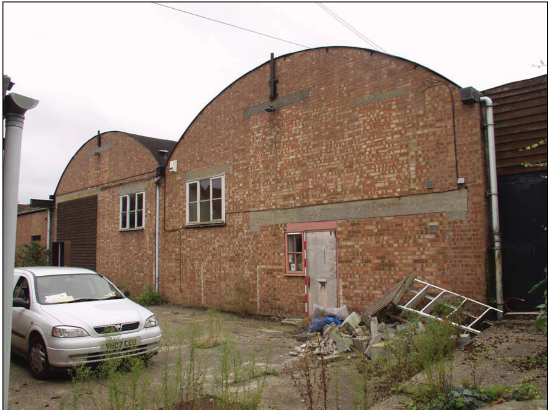
Plate 1 East elevation of Building 1, north end, taken from the north-east (DP 04)
