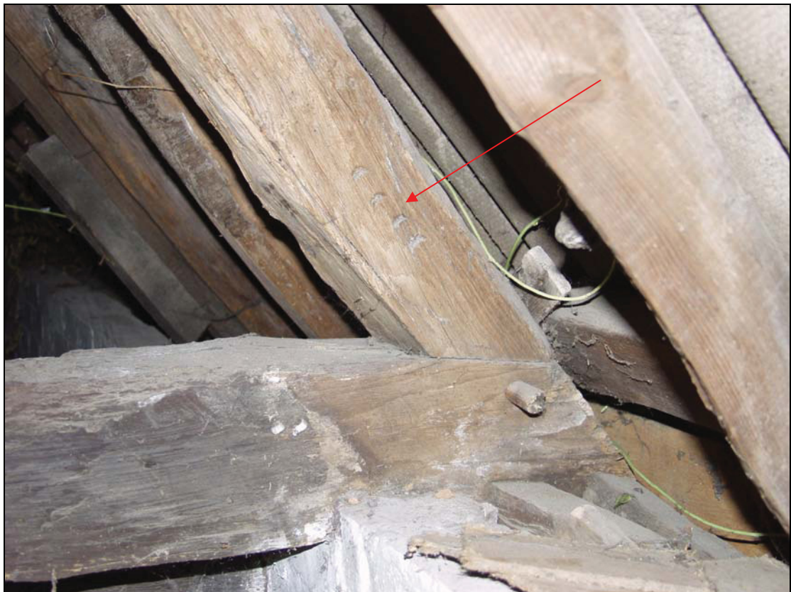
Plate 10 Detail of assembly mark on the principal rafter of the east truss, taken from the south-east (DP 29)
