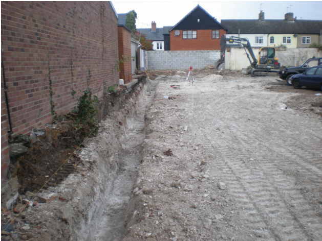
DP 3. W foundation trench. View NW.
