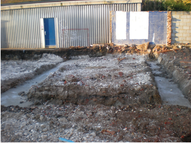
DP 7. Central part of the site. View NE.
