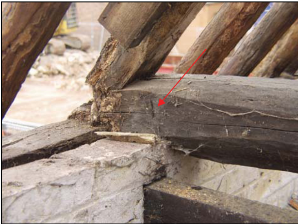
Detail of assembly mark on the south side of the tie-beam of the west truss, Building 3, taken from the north-east
