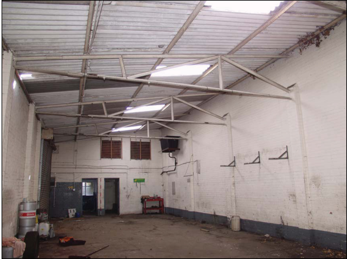
Plate 3 Unit 3 in Building 1, taken from the north (DP 10)
