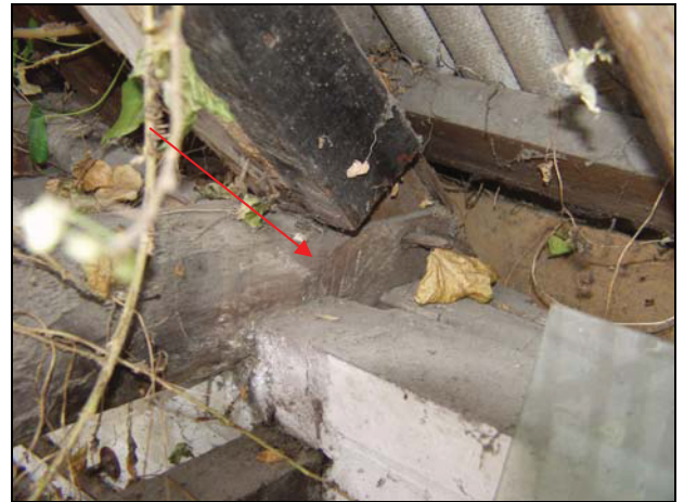
Detail of assembly mark on the north side of the tie-beam of the west truss, Building 3, taken from south-east
