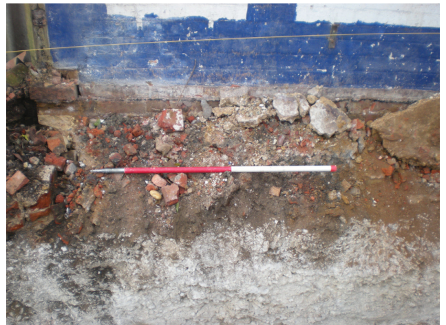
DP 6. W foundation trench. Sample section 3. View SW.
