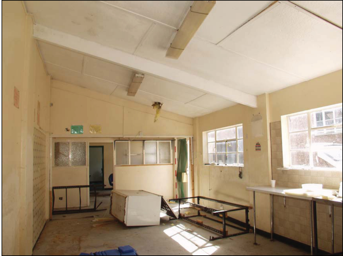
Plate 5 Interior of Building 2, northern area, taken from the north (DP 19)
