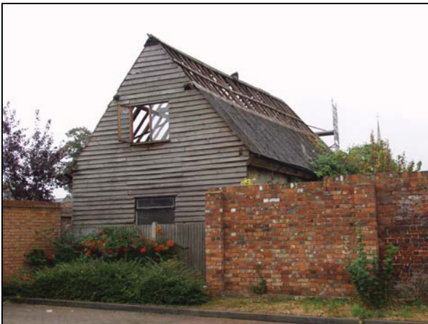
43 East elevation of Building 3, taken from the north-east
