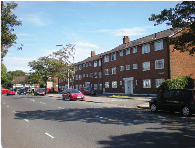
DP 1. Windmill Road and Pickering House, Ealing, London. View E.
