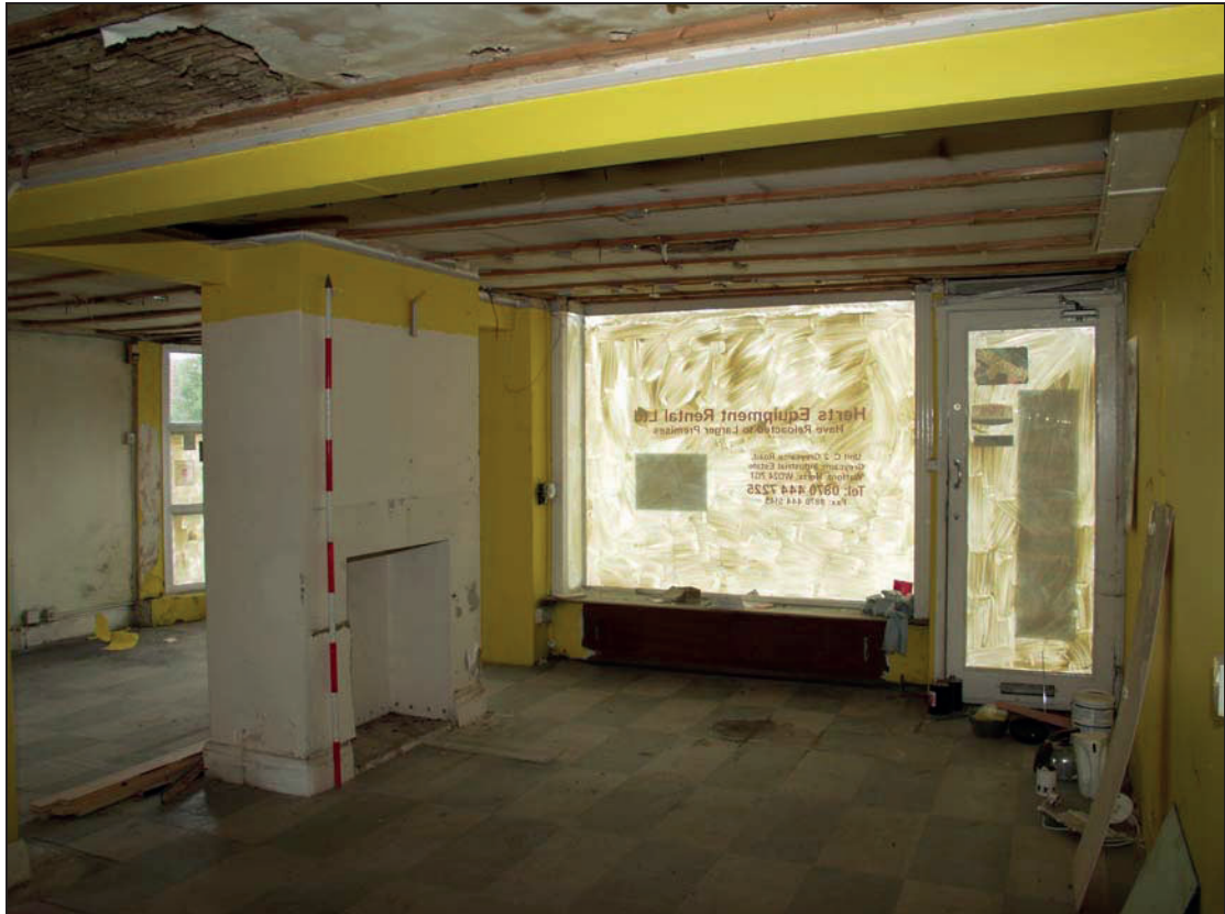
Plate 7 East side of Room 6 showing free-standing chimneystack (No. 195), taken from the south (DP 21)
