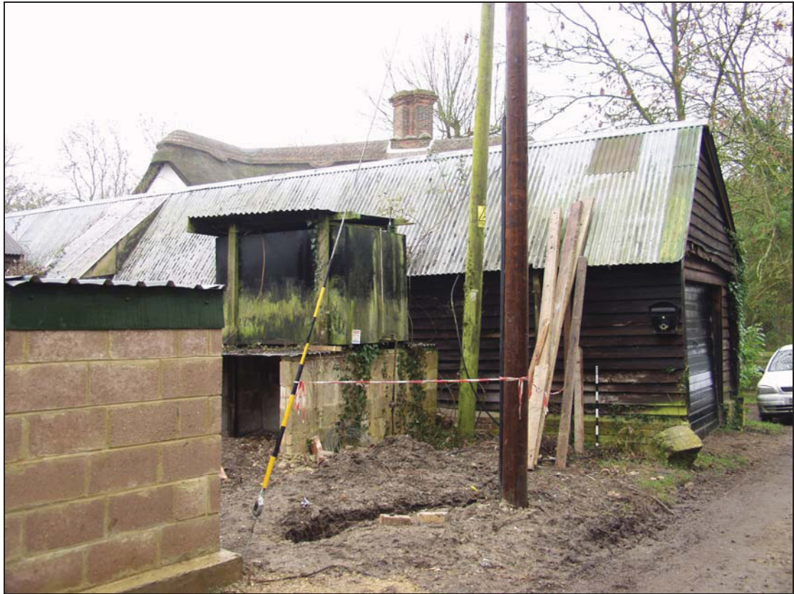
3 North elevation taken from the north-west (2)
