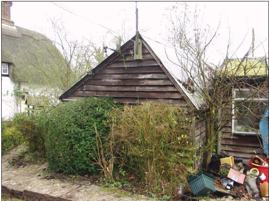
4 East elevation taken from the east (5)
