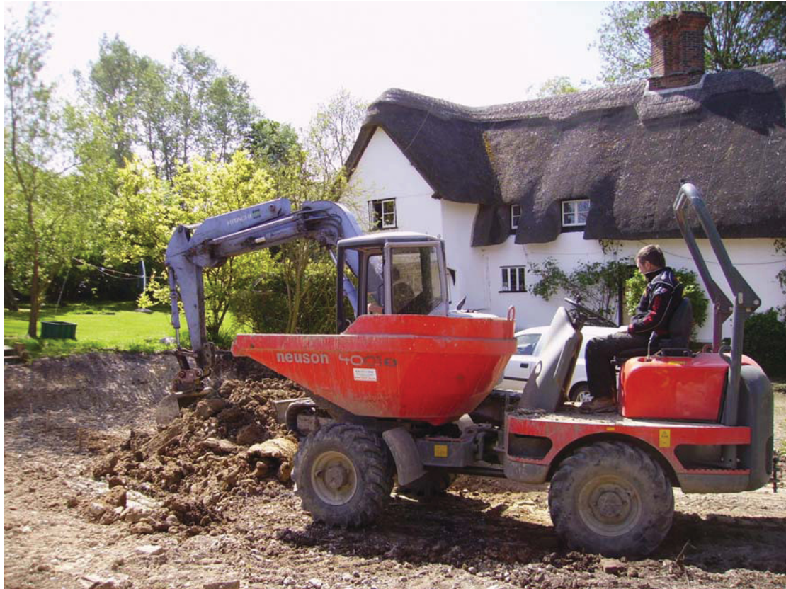
9 General view of the groundworks showing proximity to the house
