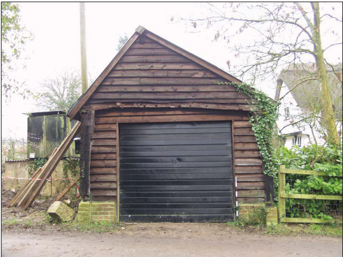
2 West elevation taken from the west (1)
