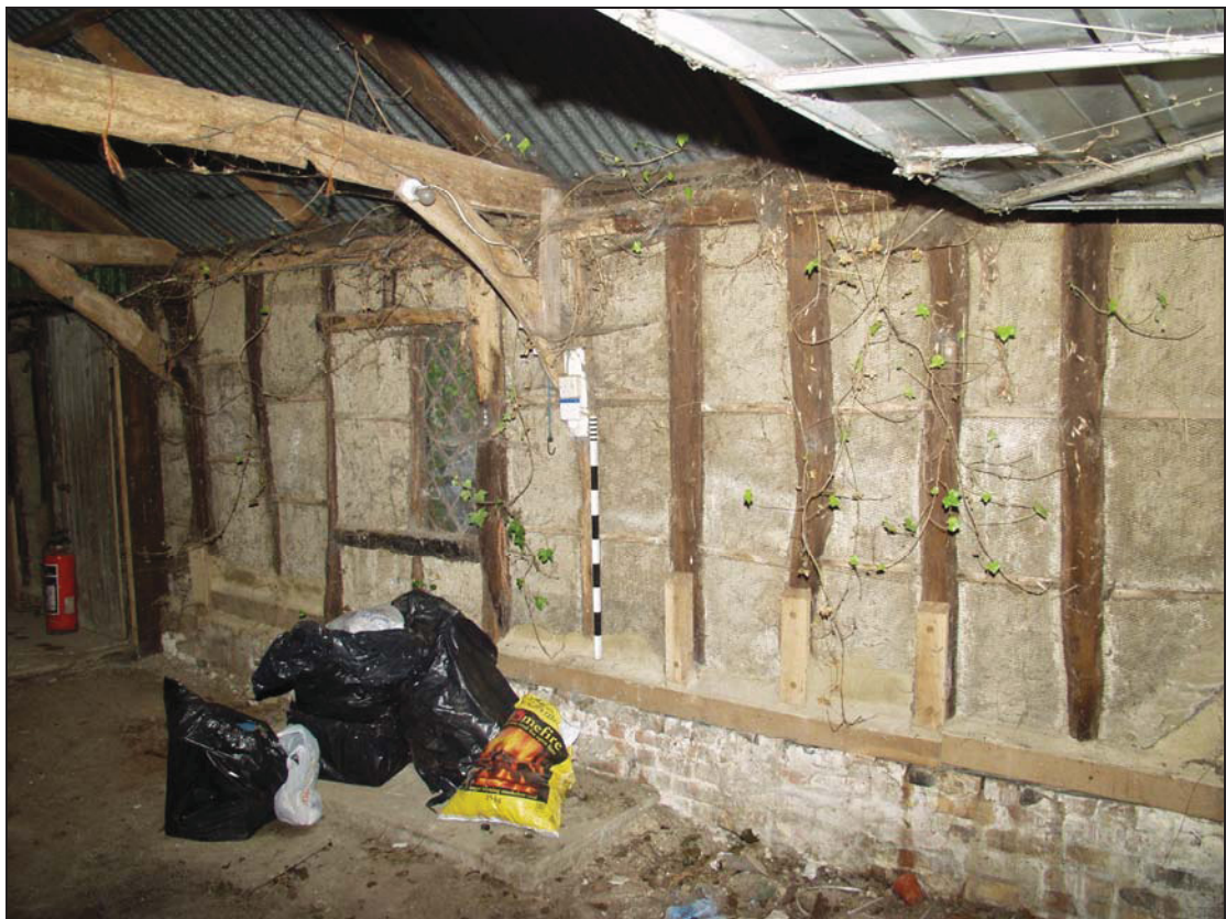
6 South walls of Bays 1 and 2, taken from the north-west (7)
