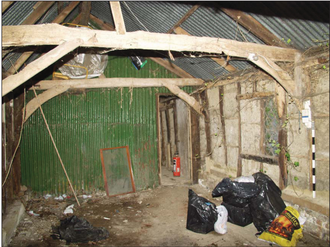
7 Intermediate trusses of Bays 1 – 2 and 3 – 4, taken from the north-west (8)
