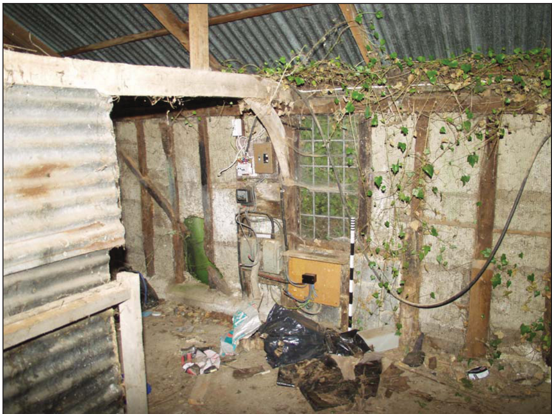
8 South wall of Bays 4 and 5, taken from the north-west (12)
