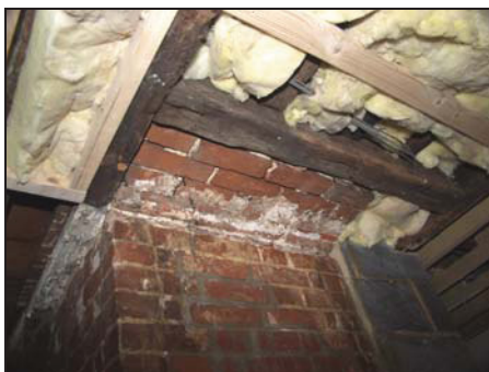
Original plaster at the rear of the chimneystack in Room 10, taken from the south-west
