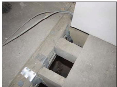
52 Exposed ceiling of Room 11 with replaced and original floor joists
