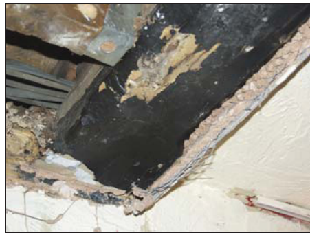
Binding joist in Room 3 showing chamfers and run-out stops, taken from the south-east
