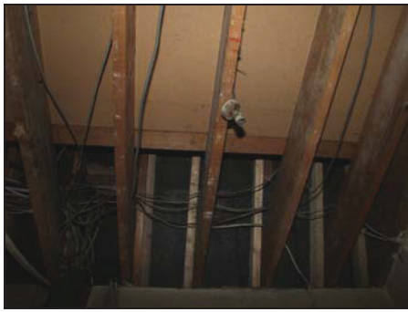
Earlier rafters alongside modern rafters over rear range (Room 5), taken from the east
