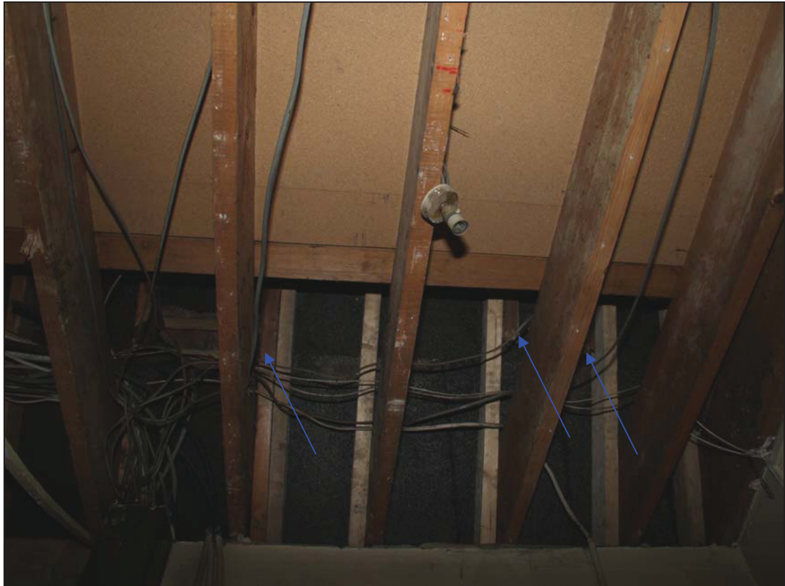
13 Earlier rafters (highlighted) alongside modern rafters over rear range (Room 5), taken from the east (37)
