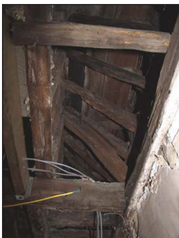
South binding joist (Room 10) showing some original and some replacement common joists, taken from the north-west
