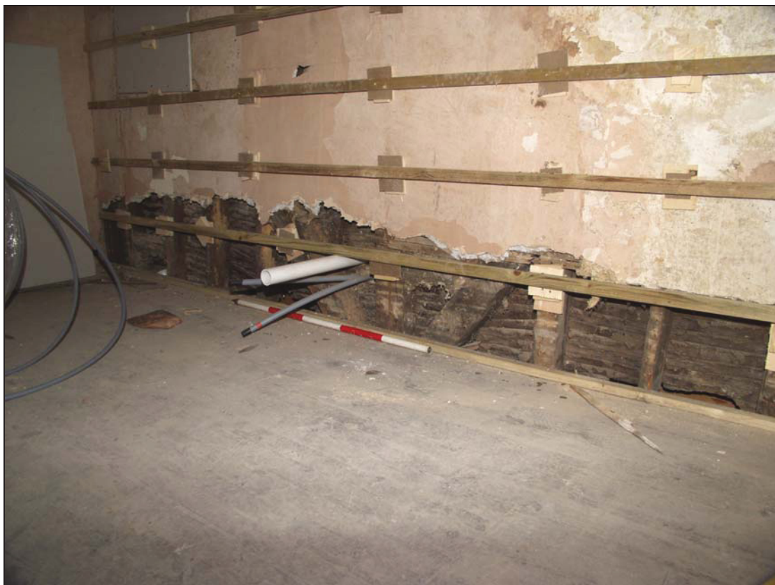
24 North wall of Room 11 (first floor of the principal range) with timber-framing visible at the base, taken from the south-east (51)
