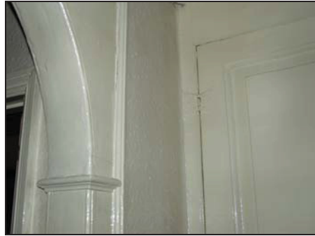
Capital on moulded jamb of archway and butterfly hinge on cupboard door, first floor landing, principal range, taken from the north-west
