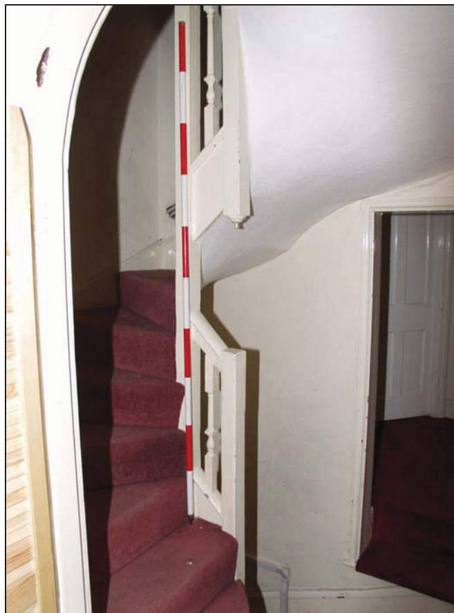
14 Dog-leg stair, first floor, principal range, taken from the south-east (16)
