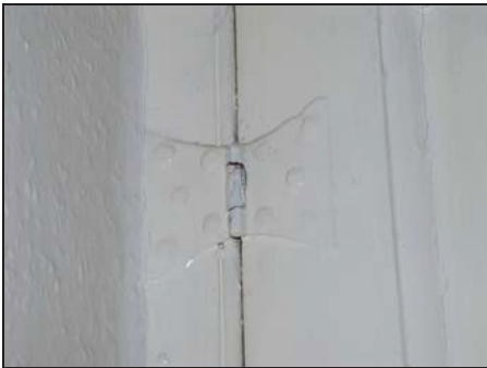
Butterfly hinge on cupboard door, first floor landing, principal range, taken from the north
