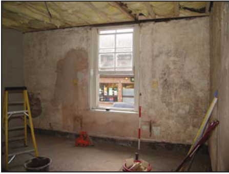
South wall of Room 10 showing exposed area of timber-framing at low level, taken from the north
