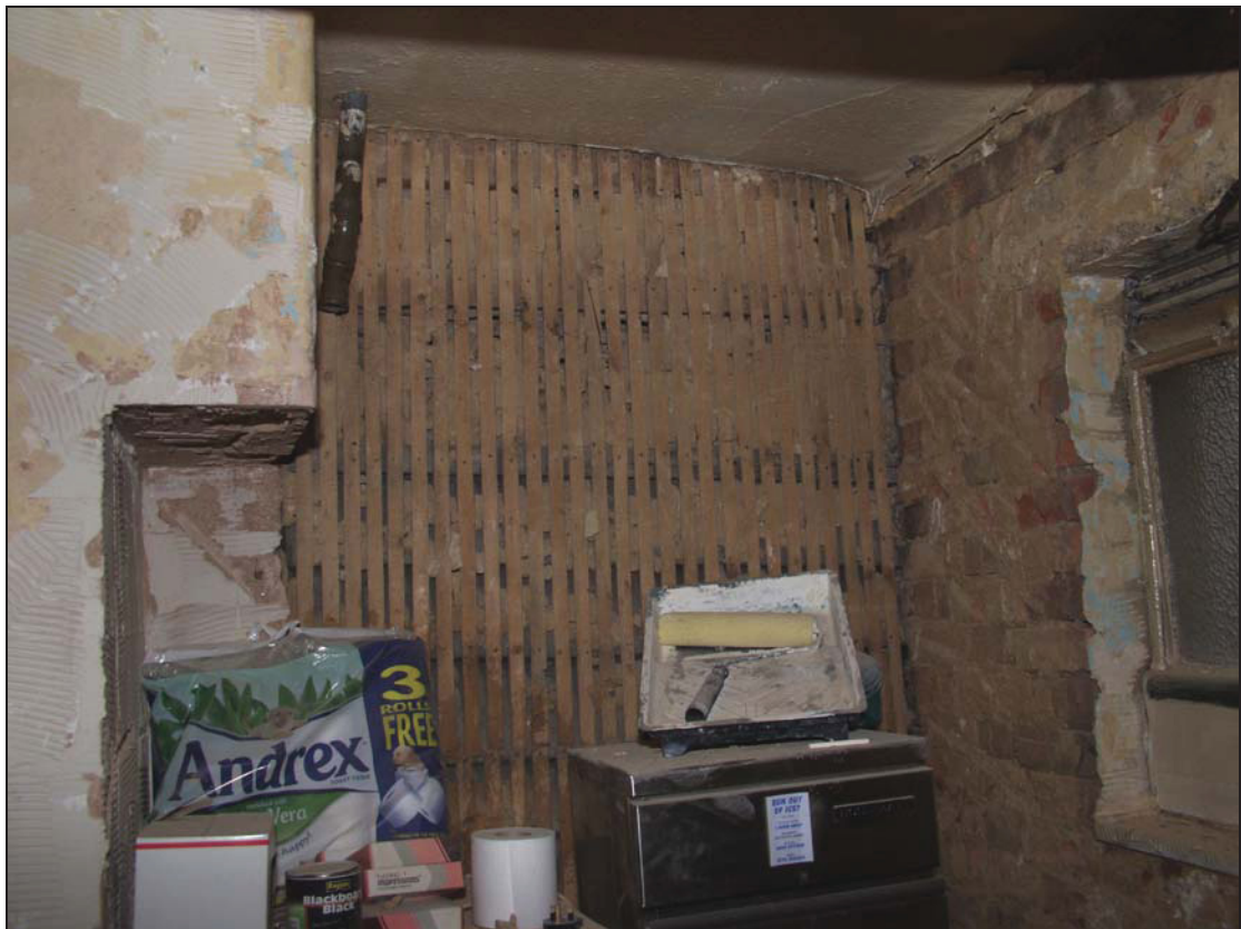
12 20 th century laths flushing over weather-boarding on north wall of principal range, taken from the north (35)
