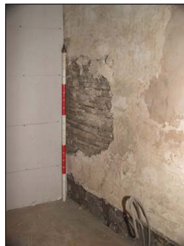
South wall of Room 10 showing exposed lath and plaster, taken from the north-west
