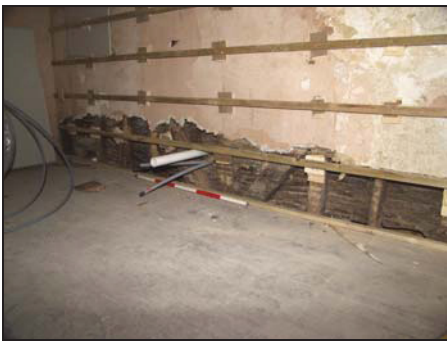
49 Detail of west wall-plate in Room 11, showing edge-halved scarf joint with metal reinforcement, taken from the east
