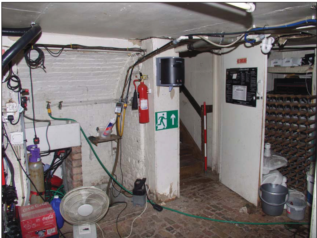
16 Corbelled brickwork to support hearth above and red brick floor in Room 6, taken from the south-west (DP 11)
