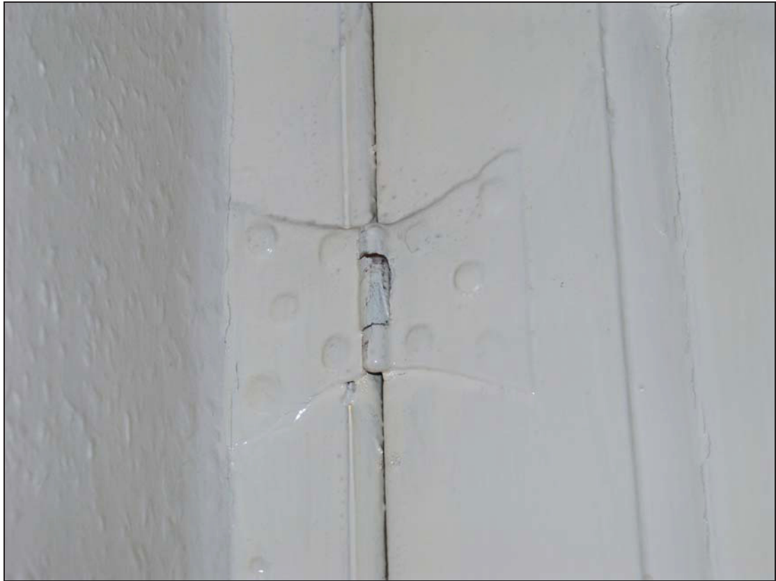
19 Butterfly hinge on cupboard door, first floor landing, principal range, taken from the north (21)
