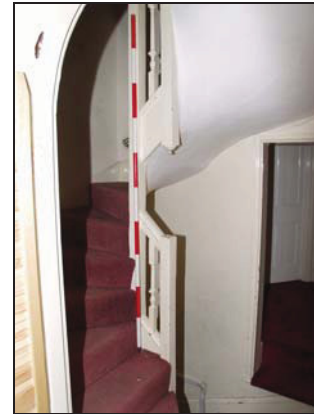
Dog-leg stair, first floor, principal range, taken from the south-east
