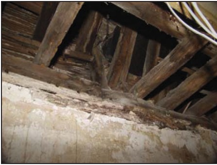
49 Detail of west wall-plate in Room 11, showing edge-halved scarf joint with metal reinforcement, taken from the east
