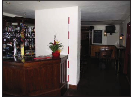
Free-standing 18 th century chimney stack between Rooms 2 and 3, principal range. Taken from the south
