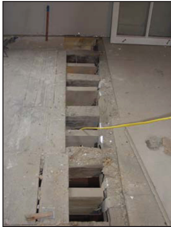
55 Exposed floor joists in Room 11 showing assembly markings, taken from the west
