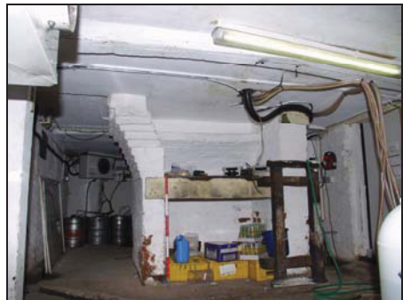
Room 7, showing jambs and corbelled brickwork for chimney and hearth above, taken from the south
