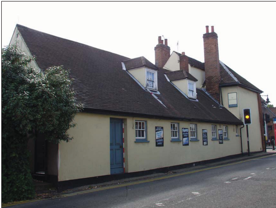
2 West elevation of rear and principal ranges with stair tower just visible between the two 18 th century chimney stacks, taken from the north-west (5)
