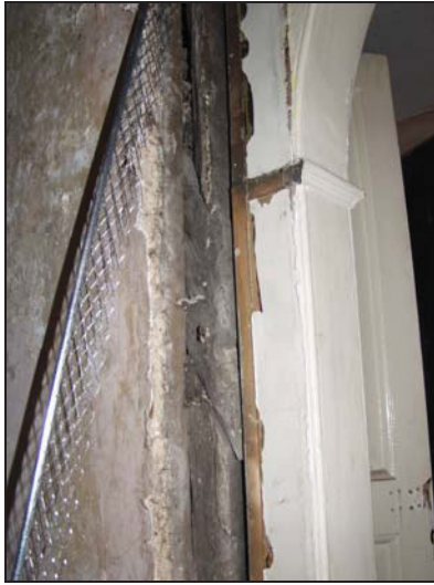
Detail on south side of entrance to Rooms 10 and 11 showing possible truncated primary brace, taken from the north-east
