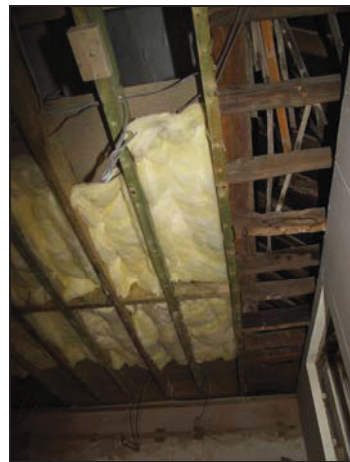
52 Exposed ceiling of Room 11 with replaced and original floor joists
