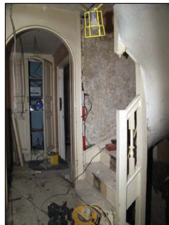
60 View of first floor landing during refurbishment, taken from the north
