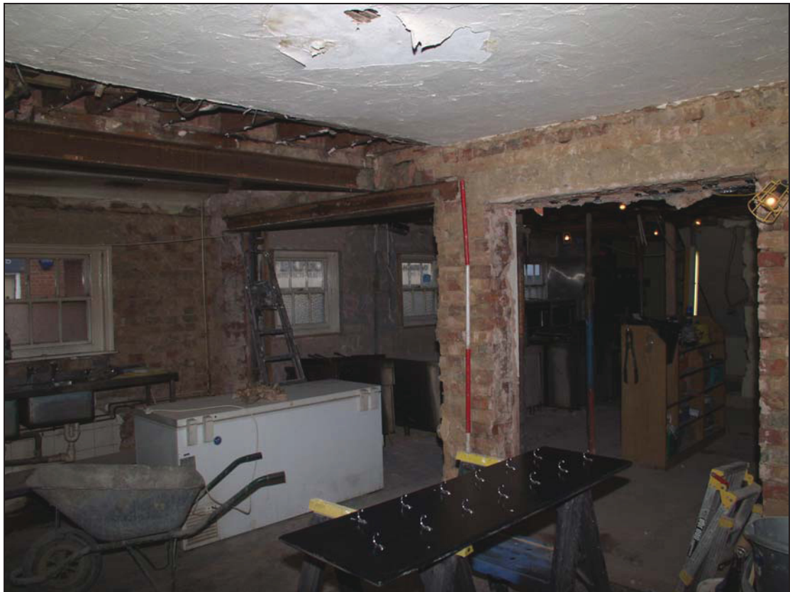
10 Twentieth century Fletton brick addition (Room 4), taken from the south-east (34)
