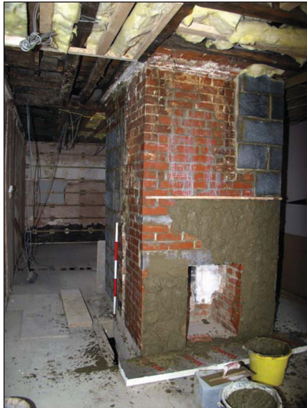
22 South face of free-standing chimney stack (first floor of principal range), taken from the south-west (40)
