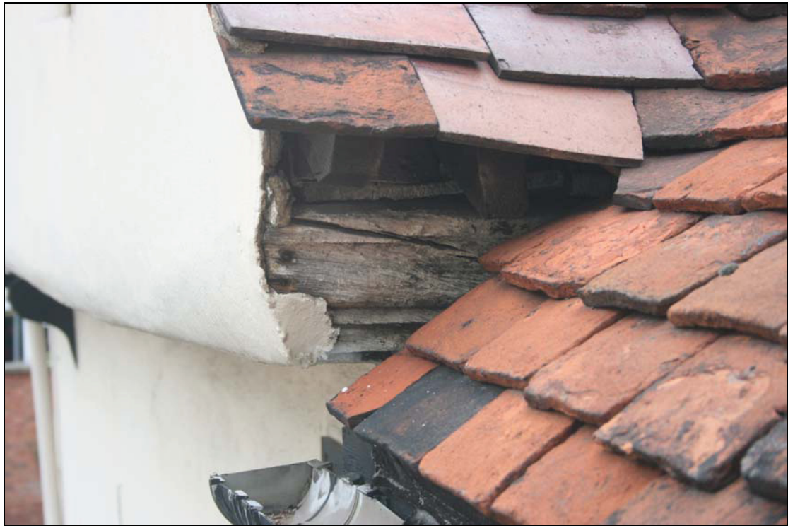
Plate 3 View of the jettied south gable of the rear range with moulded bressummer, taken from the east (DP 52)
