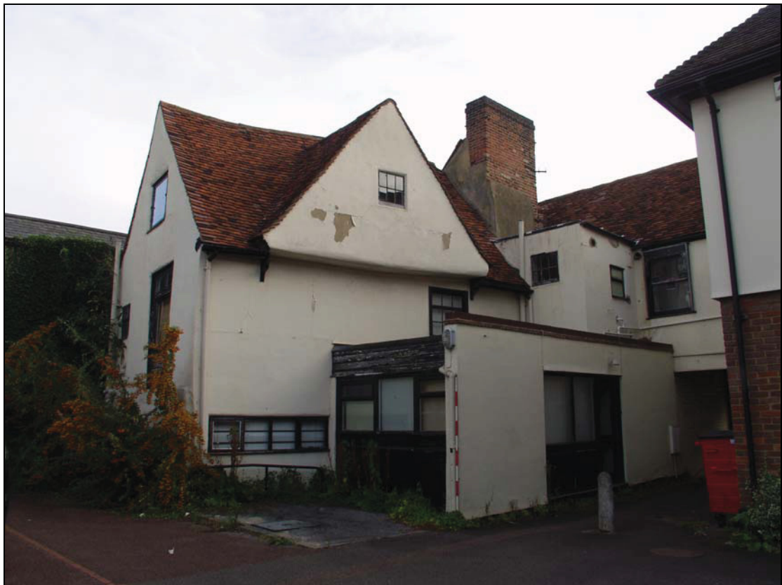
Plate 2 View of the rear range with south gable and later extensions, taken from south-west (DP 01)
