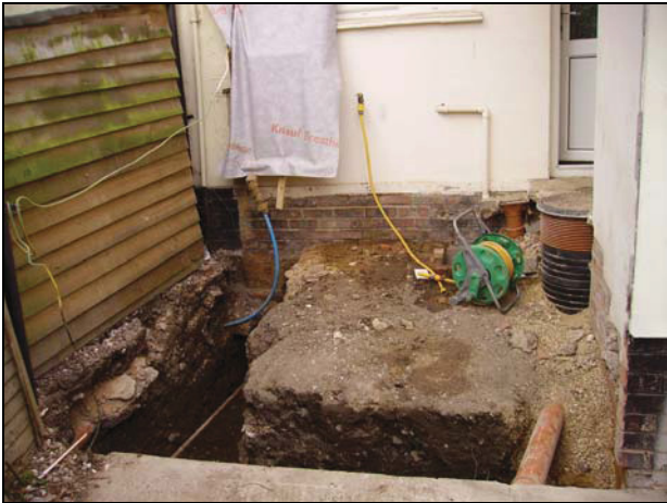
3 General view of foundation trenches, looking north.
