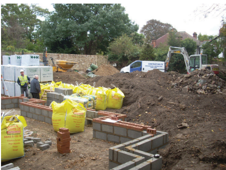
5. General site shot, facing south
