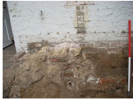
2. Sample Section 2, facing north
