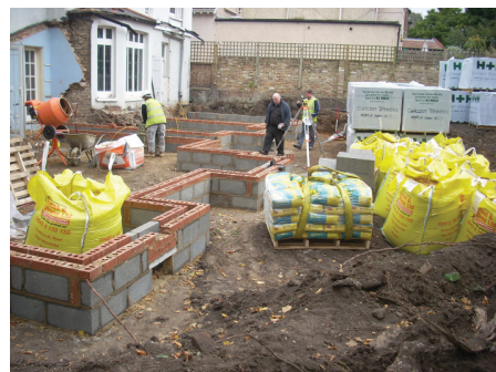
6. General site shot, facing east
