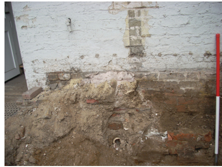
2. Sample Section 2, facing north
