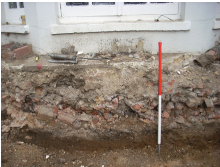
3. Sample Section 3, facing north
