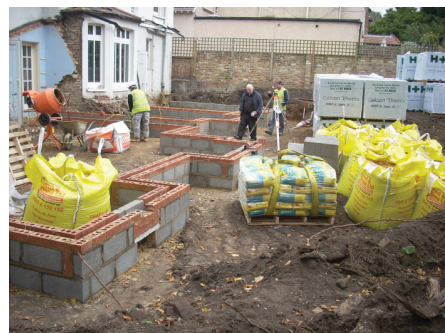
6. General site shot, facing east
