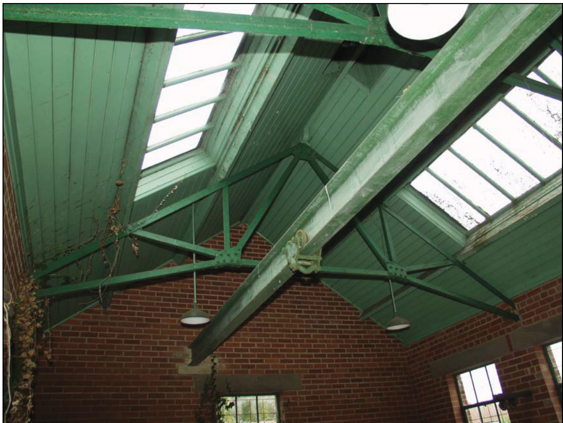
Plate 3 Roof structure of the building showing the lateral rail system, taken from the south (DP 08)
