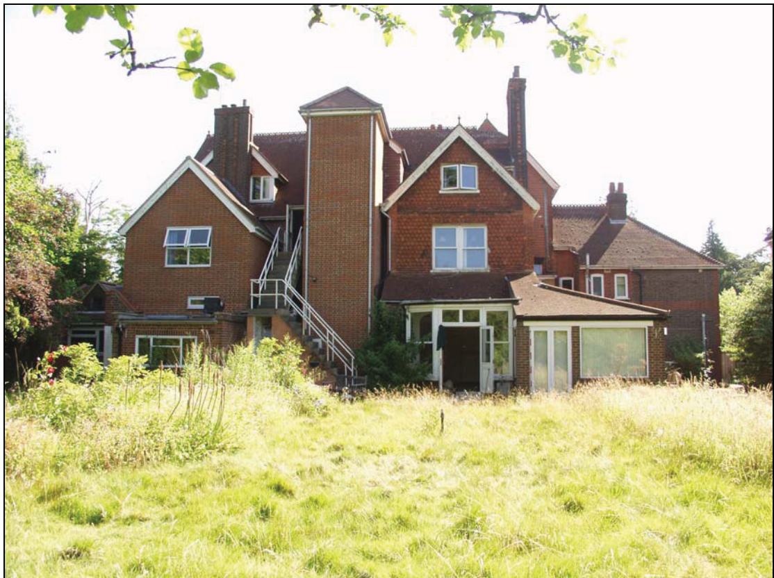
Plate 2 Rear west façade of the building with later additions, taken from the west (DP 5)
