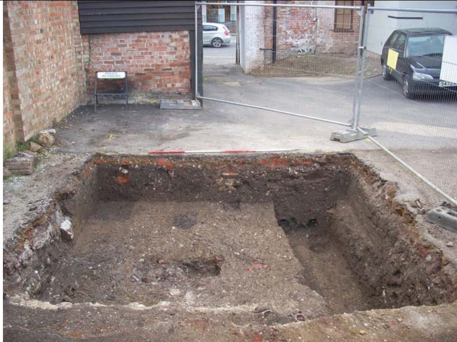
DP6 Trench 3: mid-excavation, view W
