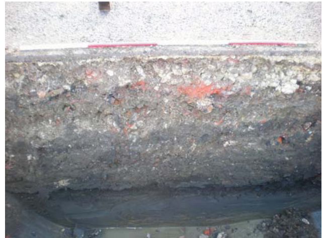
DP 8. Trench 2, NE end. Sample section. View SE.
