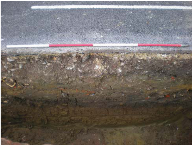
DP 15. Trench 3, NE end. Sample section. View NW.
