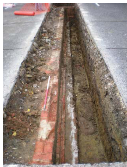
DP 12. Trench 3. View SW.
