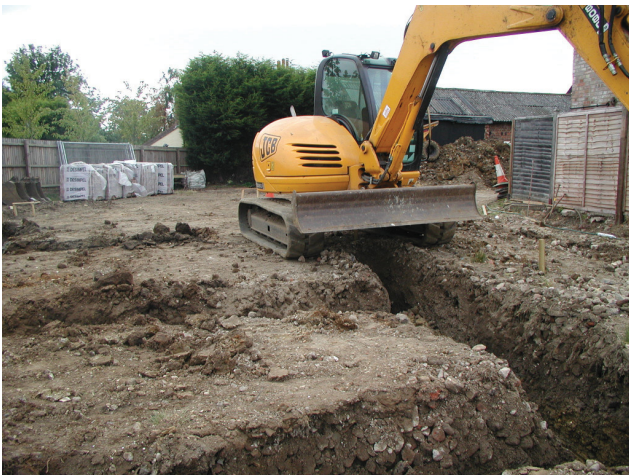
DP 3. Plot 1, the groundworks. View SW.
