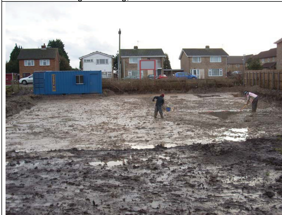
Plate 2: Site under excavation, view S towards higher ground
