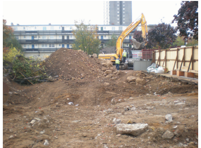
DP 2. W part of the site. View SSE.
