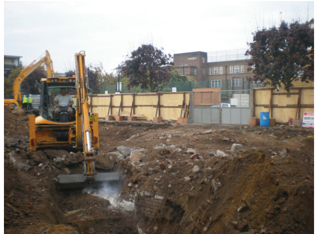
DP 4. Trial trenching, N part of the site. View S.
