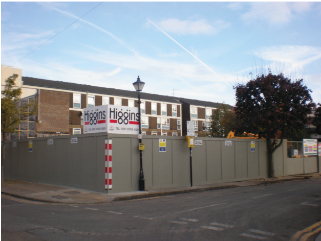
DP 1. John Bond House site, 20 Wright's Road, Bow, London. View SE.
