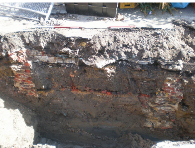
DP 5. Trench 1, N end. Sample section. View NE.
