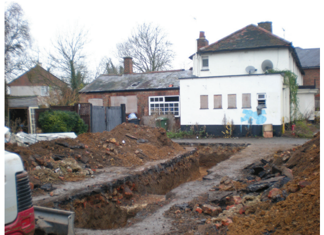
DP 2. The site. View WNW.
