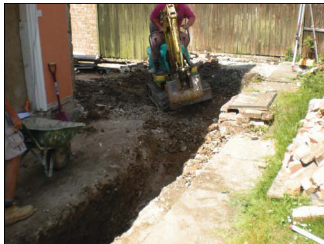
DP 6. Excavation of foundation trench, NW corner. Taken from E.
