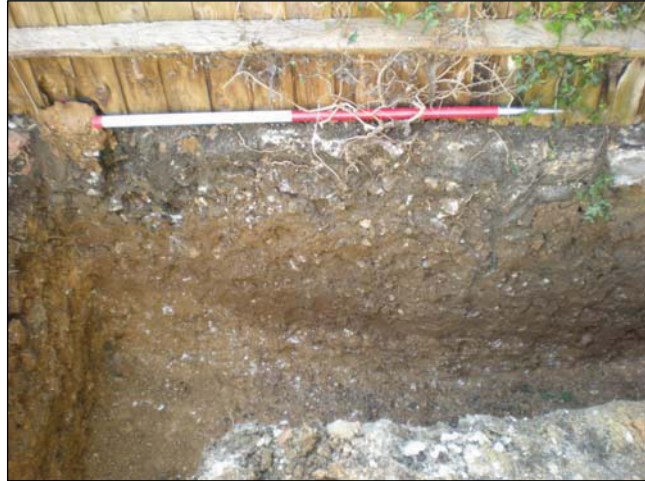
DP 4. Foundation trench to the rear of the house, SE corner. Sample section 1. Taken from WNW.
