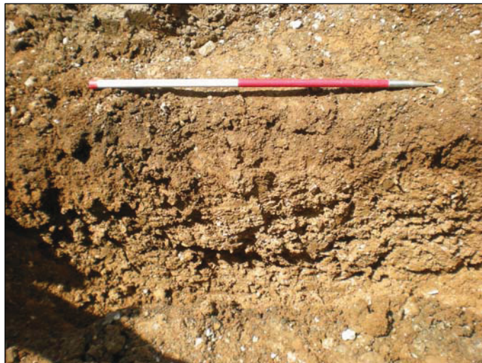
DP 10. Foundation trench to the W of the house. Sample section. Taken from ESE.
