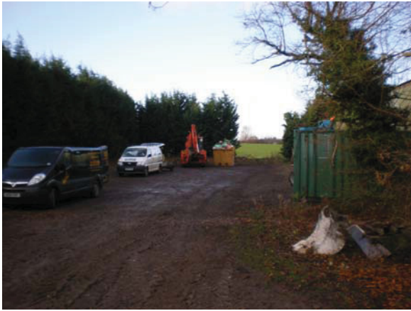
DP 1 General view of the site before work commences, looking west.
