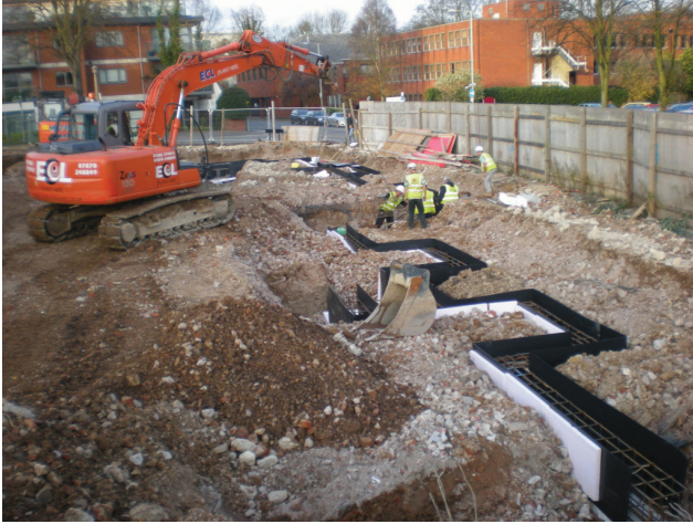
DP 7. Central/E part of the site. View NNE.
