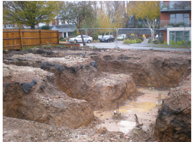
DP 2. NW corner of the site. View NNW.
