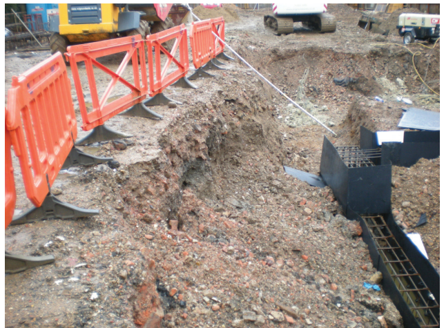
DP 12. S part of the site, foundation trench. View N.
