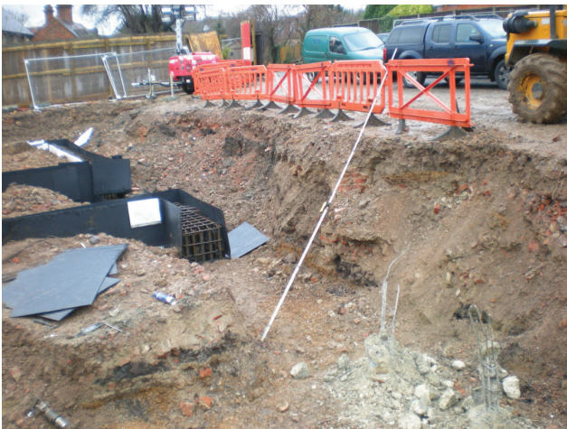
DP 11. S part of the site, foundation trench. View SSW.
