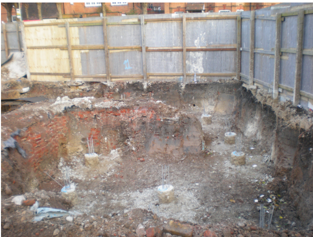
DP 9. SE corner of the site. View E.
