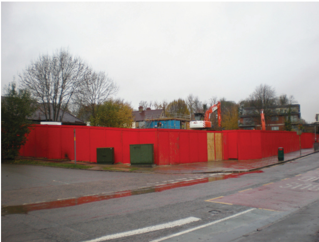
DP 1. 10-12 High Street, Rickmansworth, Hertfordshire. View NNW.
