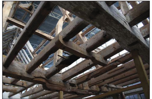
Ceiling of the central bay in Room 5 showing position of lost pulley wheel system, taken from the south-west
