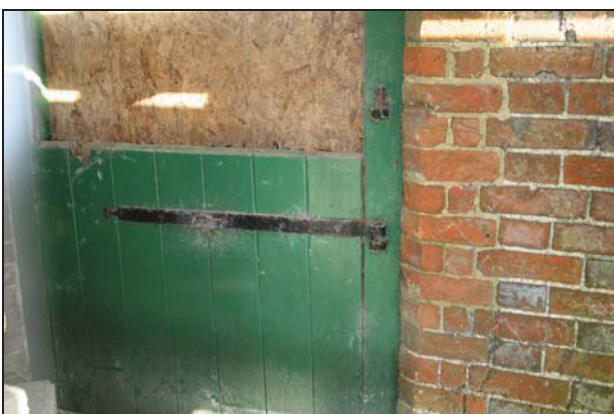
Strap-hinge on the west door of the main range, ground floor, taken from the west
