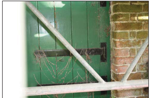
Strap-hinge on west door of the granary, ground floor, taken from the west
