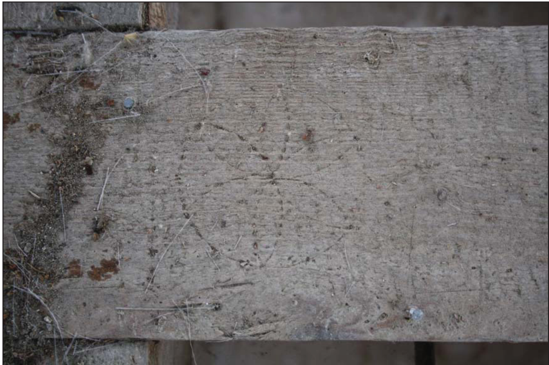
Plate 7 Detail of daisy-wheel scribed onto a ceiling joist in the main range, upper floor, taken from above (DP 71)
