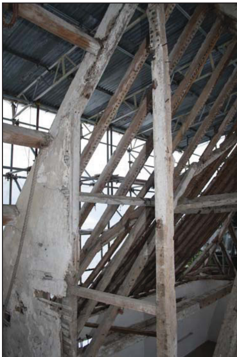
Detail of former partition and doorway in the roof space between the main range and the cross-wing, taken from the south-east
