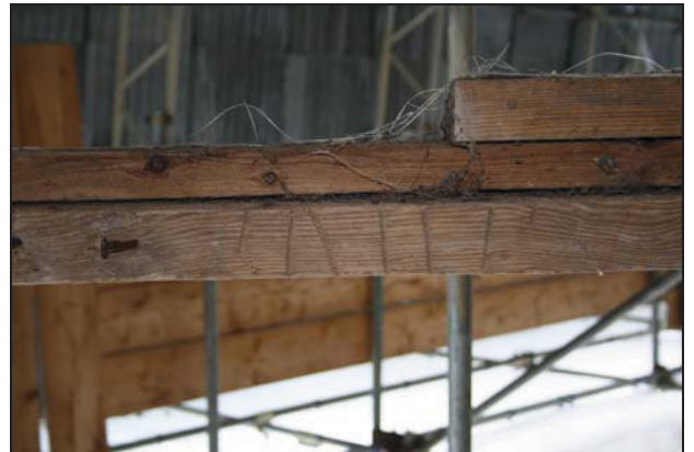
Detail of bracing mark on a rafter in the cross-wing, taken from the north
