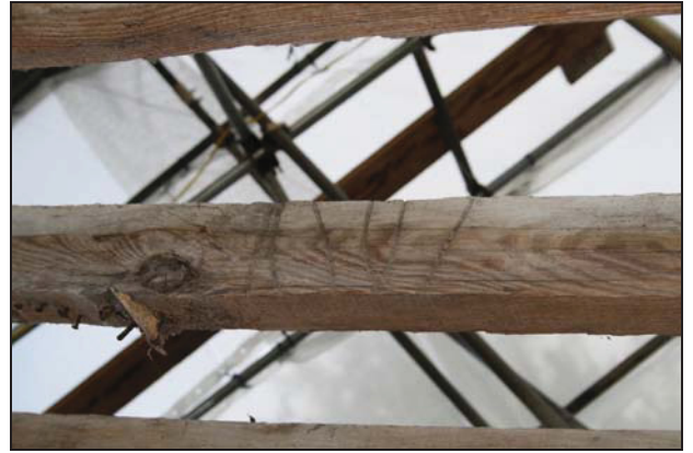
Detail of bracing mark on a rafter in the cross-wing, taken from the south
