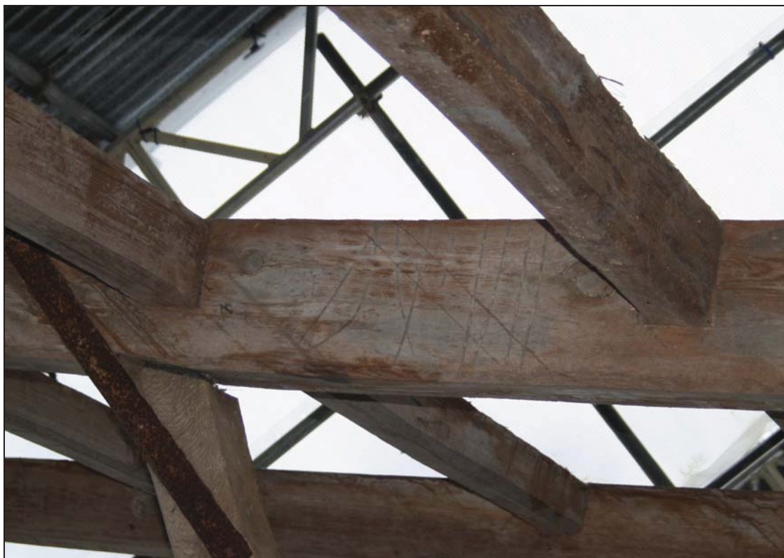
Plate 6 Detail of bracing mark on principal rafter of the main range, taken from the north (DP 69)
