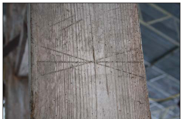
Detail of the setting-out mark on a rafter in the roof of the main range, taken from the south
