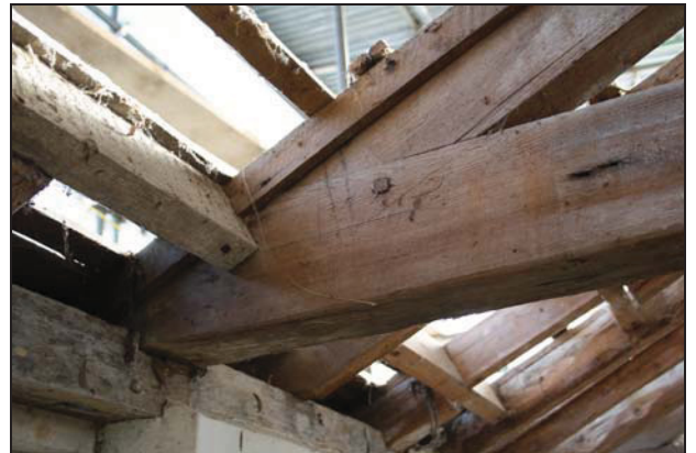
Detail of scribing marks on the south truss of the granary, taken from the north
