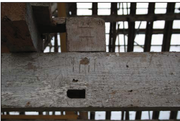
Detail of tie-beam and stump of queen strut in the cross-wing, taken from the east
