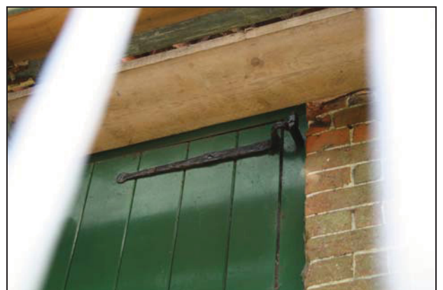
Strap-hinge on the west door of the main range, taken from the west
