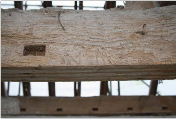
Detail of bracking mark on tie-beam of the cross-wing, taken from the east
