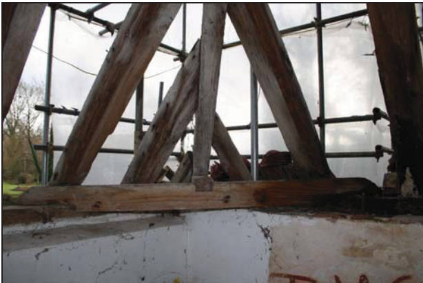
Detail of an angle-tie in the roof of the cross-wing, taken from the north-west
