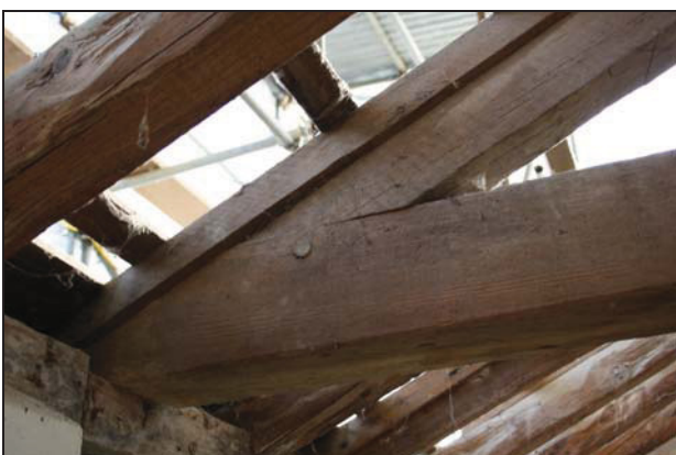
Detail of scribing marks on the north truss of the granary, taken from the north
