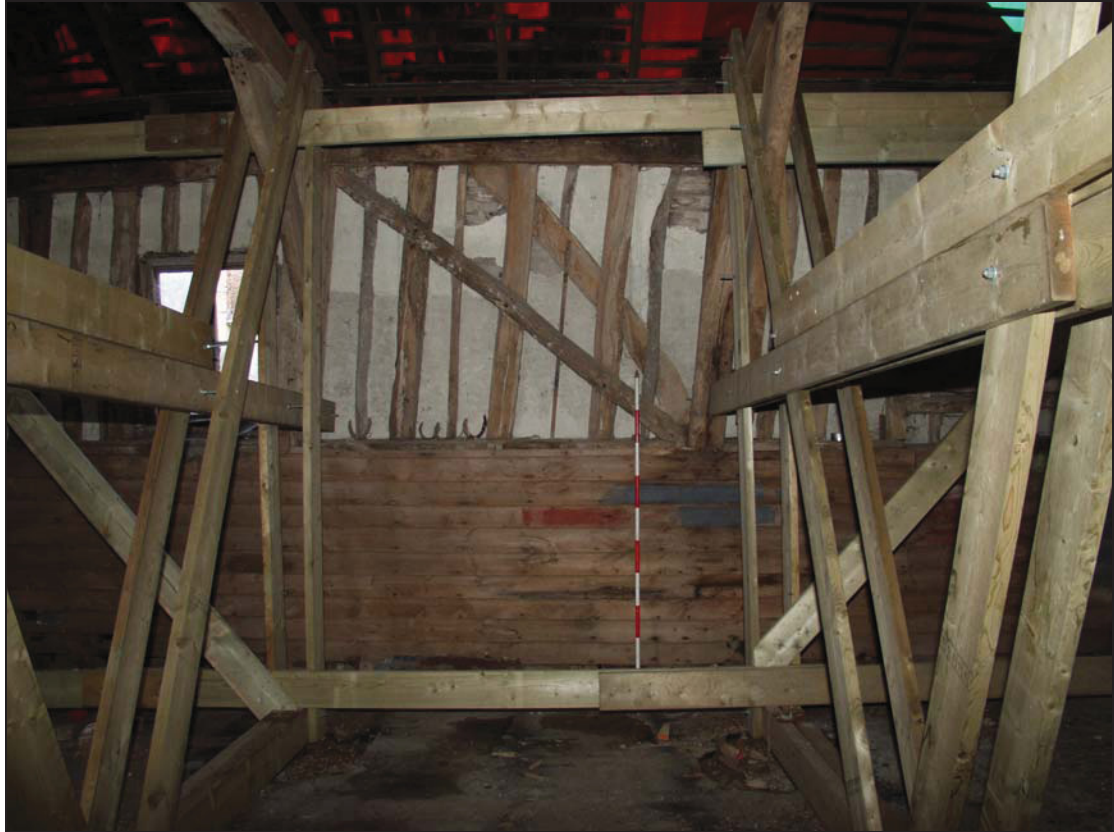
Plate 3 West wall of Bay 7 showing typical wall panelling, Building 1, taken from the east (DP 53)
