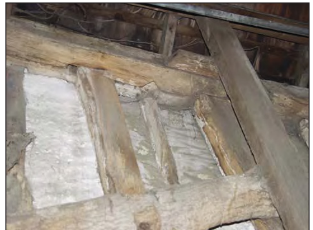
Internal face of the west post of Truss 5 showing wattle notches for an intermediate partition, taken from the south-east
