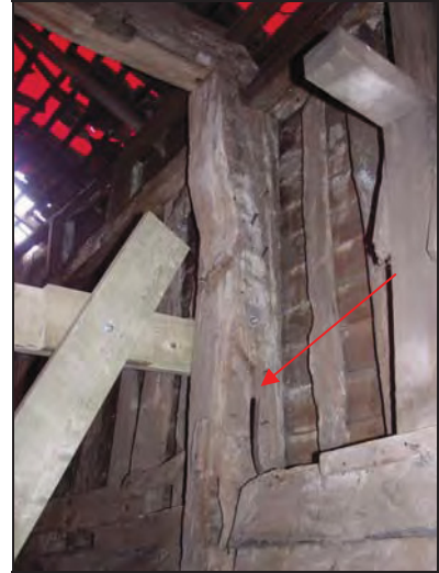
92 East post of Truss 2 showing brace mortice (indicated), Building 1, taken from the south-west
