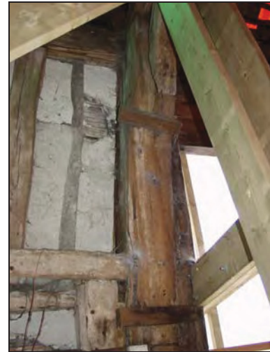
Detail showing wattle notches in the west post of Truss 7 (indicated), Building 1, taken from the north-east
