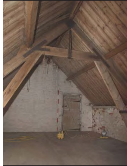
128 North side of Room 3, Building 7: upper floor, taken from the south-west
