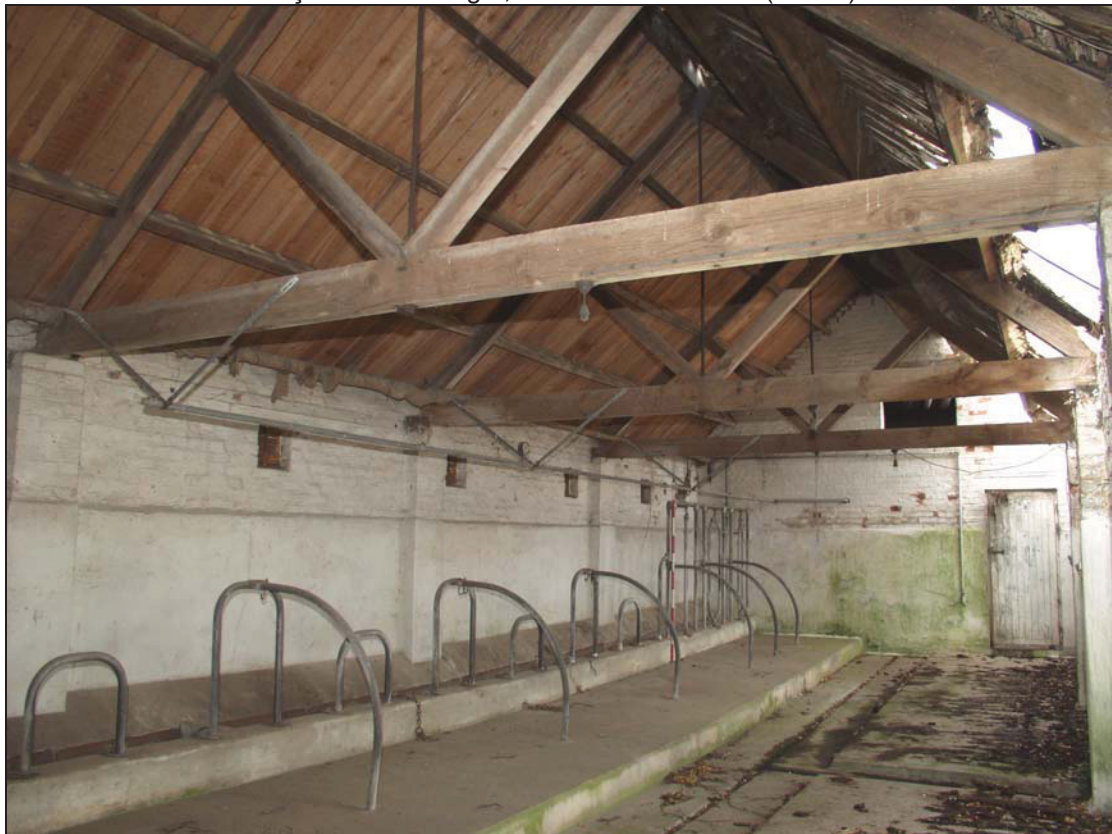
Plate 12 Interior of Building 3, taken from the north-east (DP 69)
