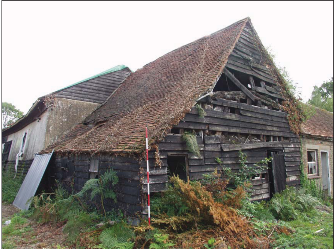
Plate 7 West and south elevations of Building 2, taken from the south-west (DP 26)
