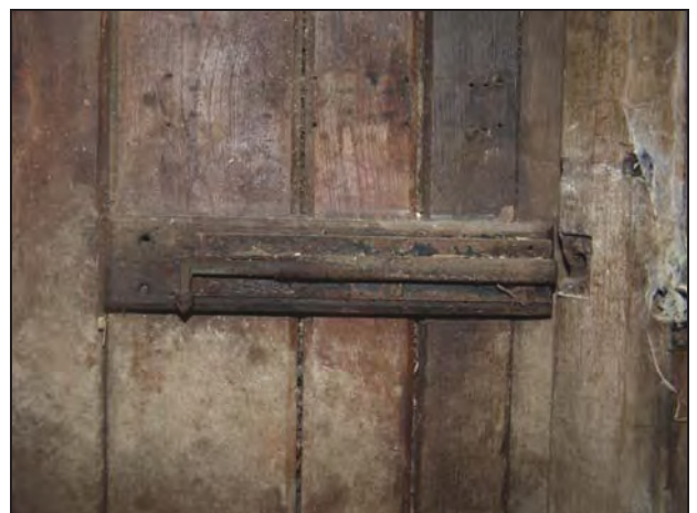
Detail of the bolt on the door to the south loosebox in the stable, Building 7, taken from the north
