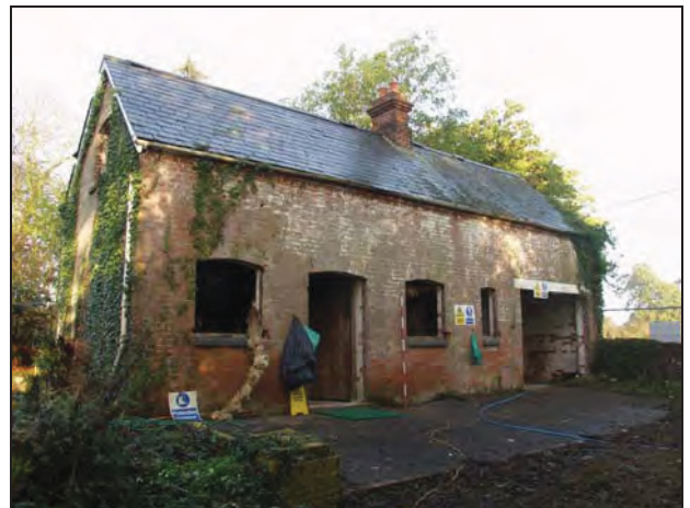
96 East elevation of Building 7, taken from the south-east
