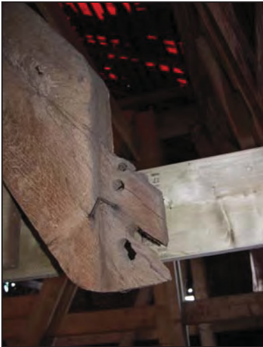
Detail of edge-halved and bladed scarf joint in the west wall-plate of Building 1, Bay 7, taken from the north-east
