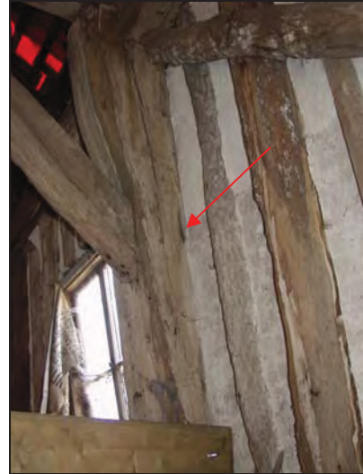
Detail showing wattle notches in the west post of Truss 7 (indicated), Building 1, taken from the north-east
