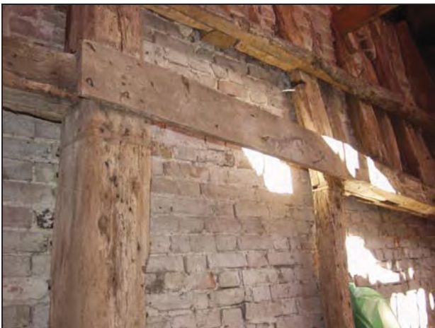
95 Detail of north gable wall of Building 1 showing prick post and adjacent stud with inserted chocks, taken from the south-west
