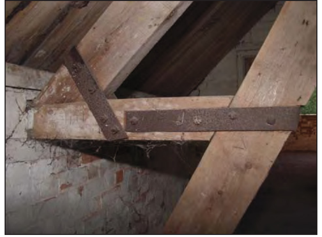
Detail on the north truss of Building 7 showing metal strapping, taken from the north
