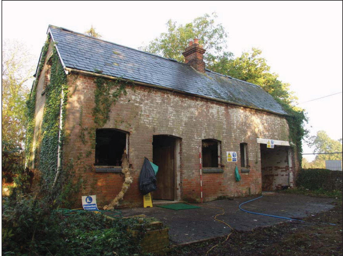
Plate 17 East elevation of Building 7, taken from the south-east (DP 96)
