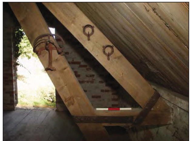
132 Detail showing equipment on the upper floor of Building 7, taken from the south
