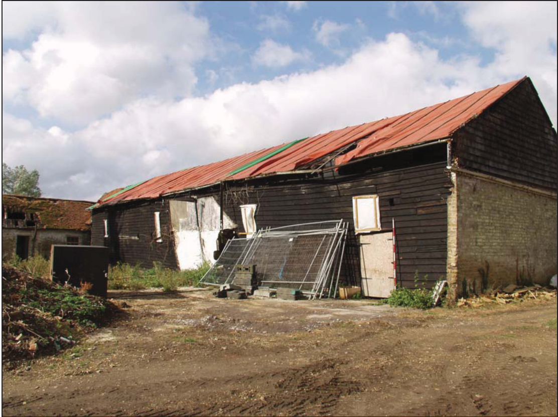
Plate 1 East façade of Building 1, taken from the north-east (DP 31)
