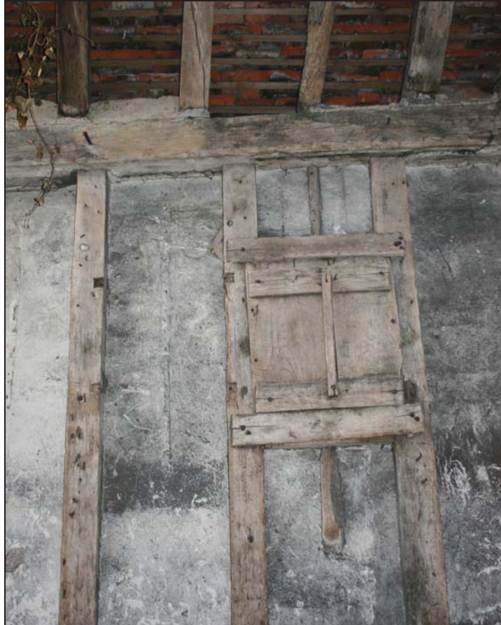
Plate 9 Detail of early window on the west wall of Building 2, taken from the south-east (DP 78)
