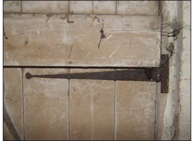
Detail of the strap-hinge on the door between Rooms 1 and 2, Building 7: upper floor, taken from the south
