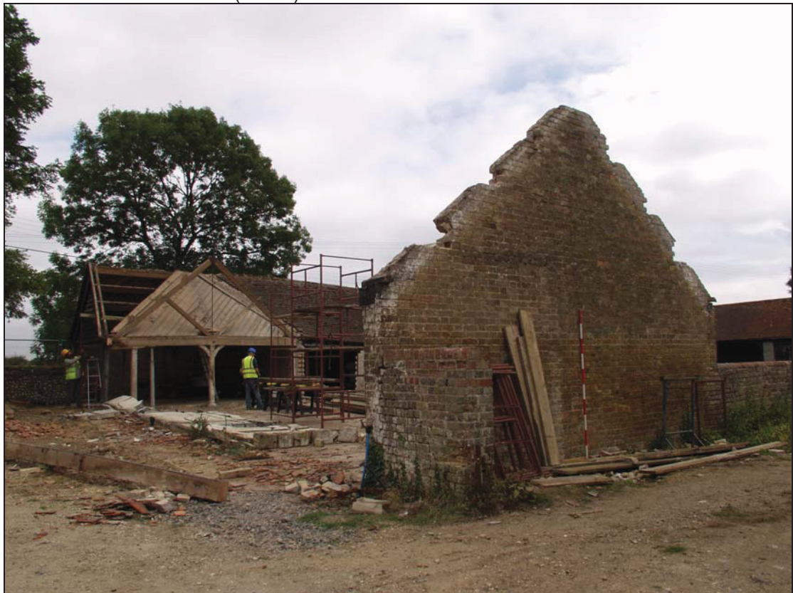
Plate 16 South and west sides of Building 6, taken from the south-west (DP 11)
