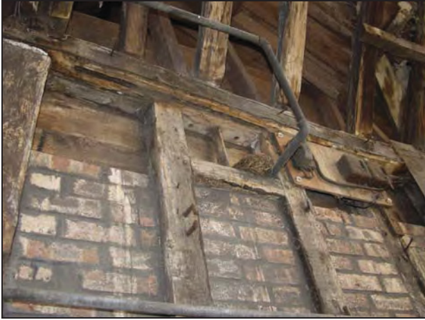
Detail of blocked early window on the east wall of Building 2, taken from the west
