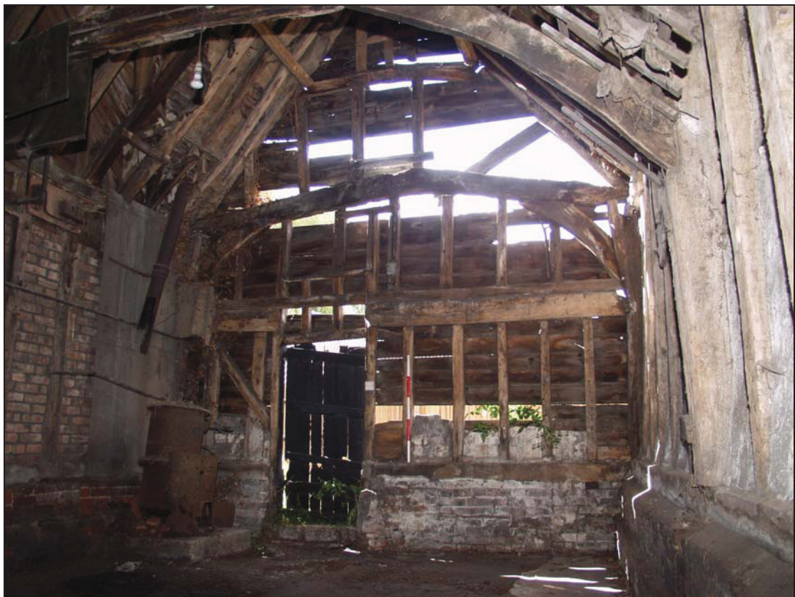
Plate 8 South gable end of Building 2, taken from the north (DP 65)
