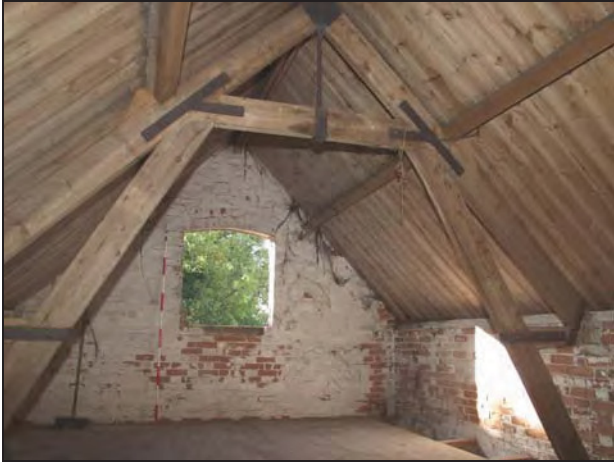
127 South side of Room 2, Building 7: upper floor, taken from the north-east
