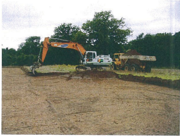
DP1. Topsoil stripping in north west corner.
