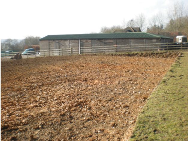
DP 3. W part of the site with ground reduced. View W.
