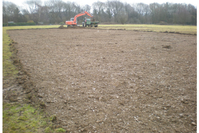
DP 2. The site with topsoil stripped. View SE.
