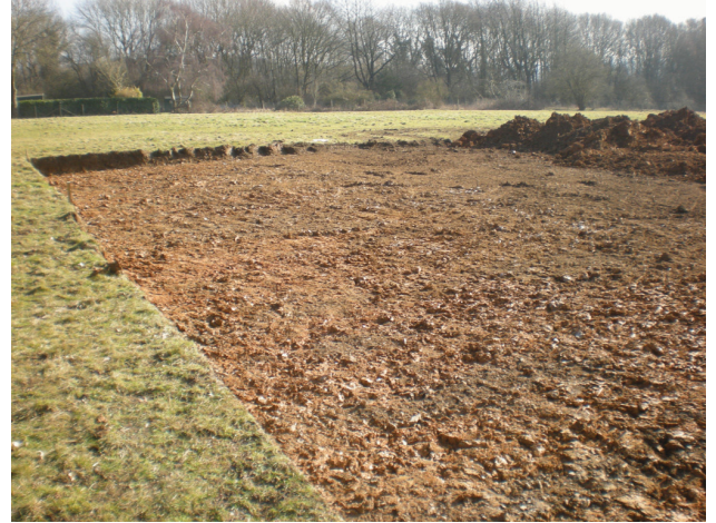
DP 4. E part of the site with ground reduced. View SE.
