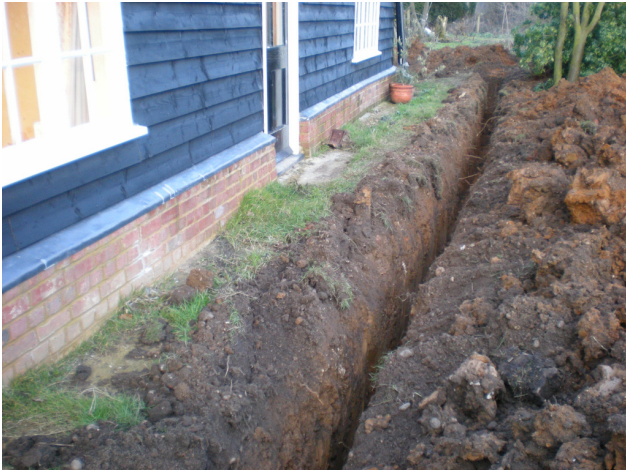
DP 3. Service trench, S part. View ENE.
