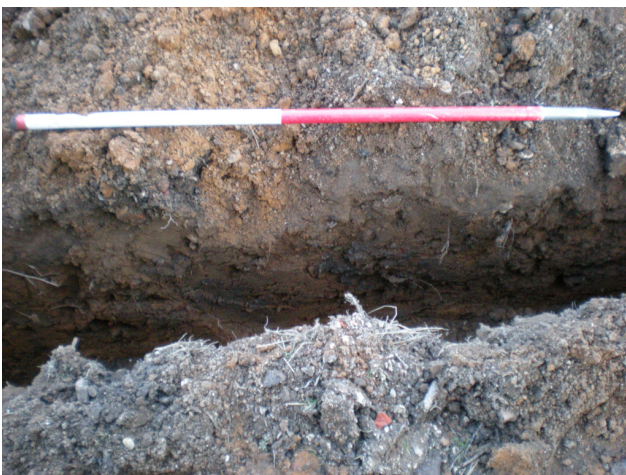
DP 5. SE part of service trench, sample section 2. View SSE.
