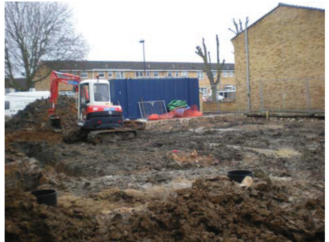
DP 2. The site. View SE.
