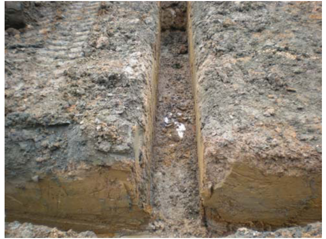
DP 4. Central foundation trench. View E.
