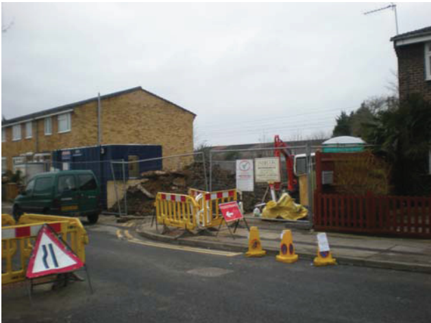
DP 1. Land adjacent to 99 Ramney Drive, Enfield EN3 6DX. View SW.
