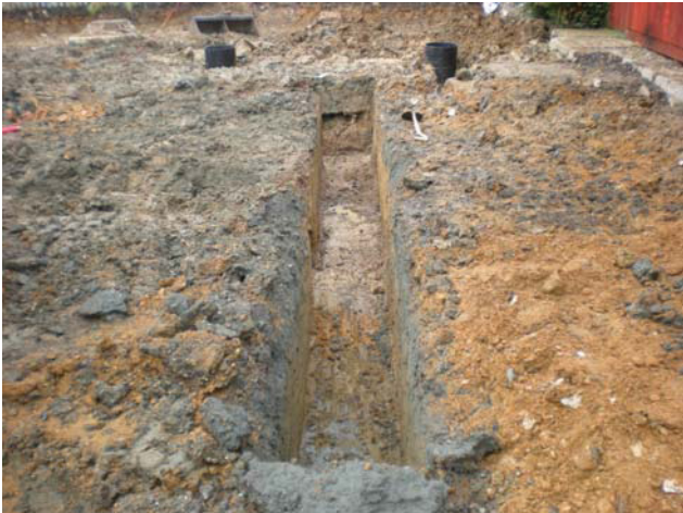
DP 3. W foundation trench. View S.
