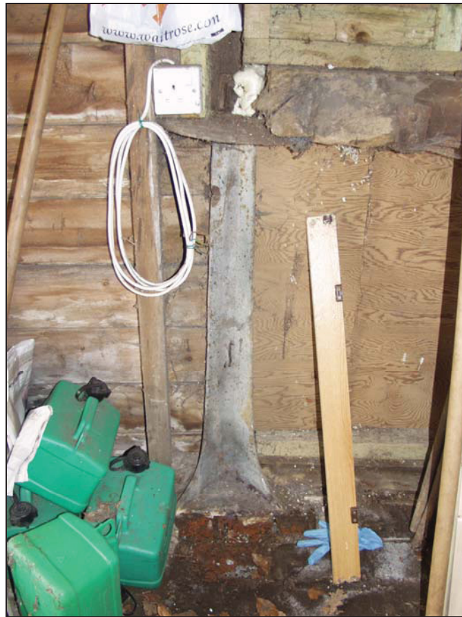
Plate 9 Detail of surviving stylobate in central unit of Building 5 (west wall), taken from the east (34)
