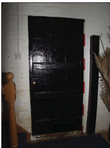
11 Door giving access to Building 3 from Building 1, taken from the south
