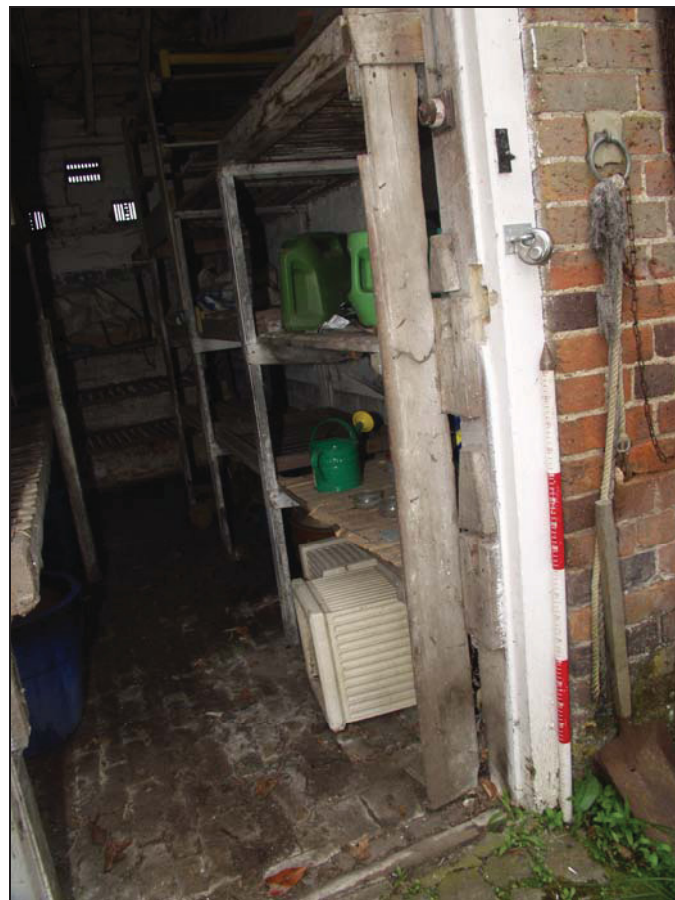
Plate 6 Detail of locking bar system to the storage unit (Building 4), taken from the south-east (26)
