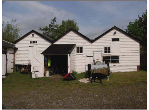
8 South elevation of Building 5, taken from the south
