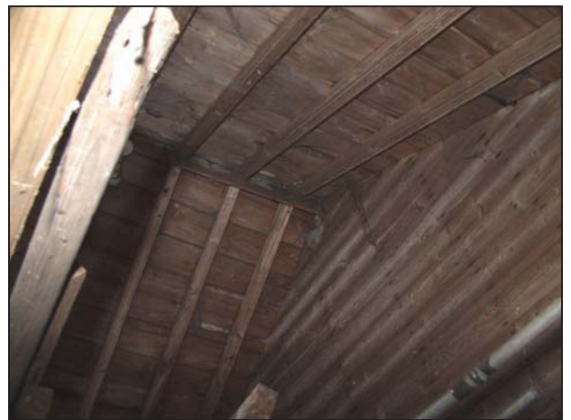
36 Roof space of east unit of Building 5, taken from the south-east
