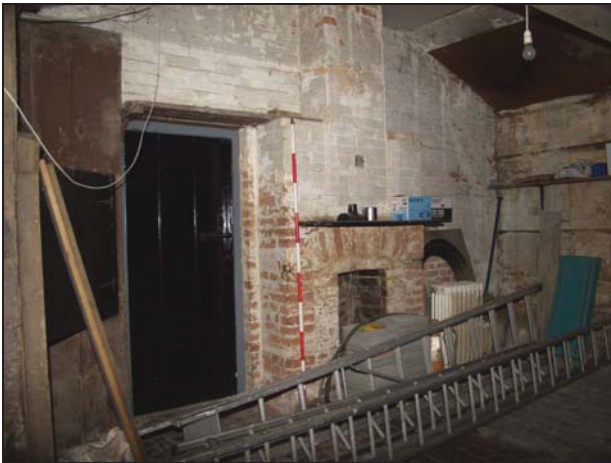
21 South wall of Building 3, taken from the north-east
