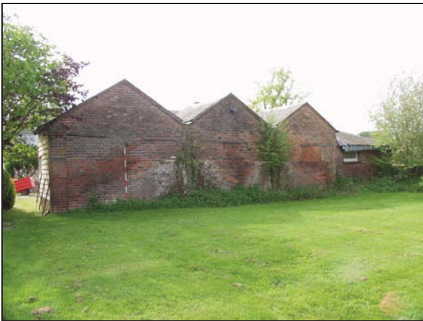
9 North elevation of Building 5, taken from the north
