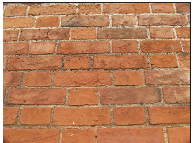
Line of queen closers (indicated) in the west wall (above level of the former garden wall) showing division between Buildings 3 and 4, taken from the west
