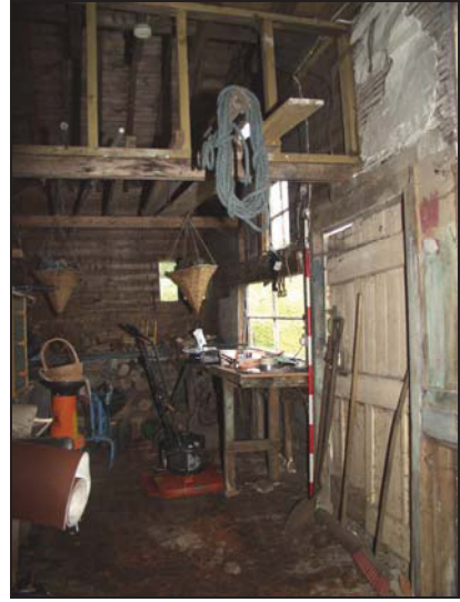
32 Interior of Building 5 (east end), taken from west
