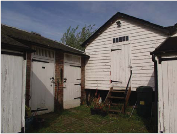
7 East elevation of Building 4 (north end) and south elevation of Building 5 (west end), taken from the south-east
