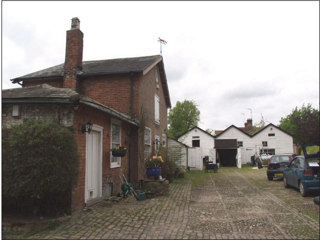
Plate 1 General view of the assessment buildings, taken from the south (39)
