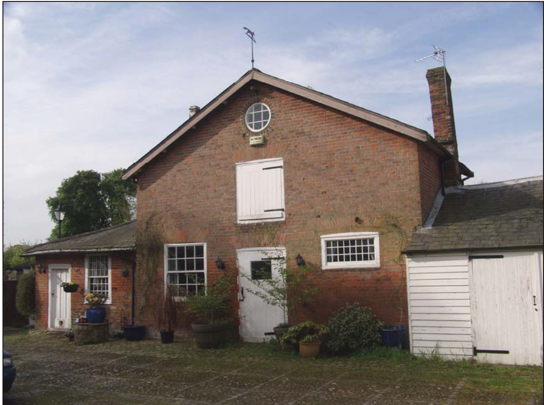
Plate 2 East façade of Building 1, taken from the east (5)
