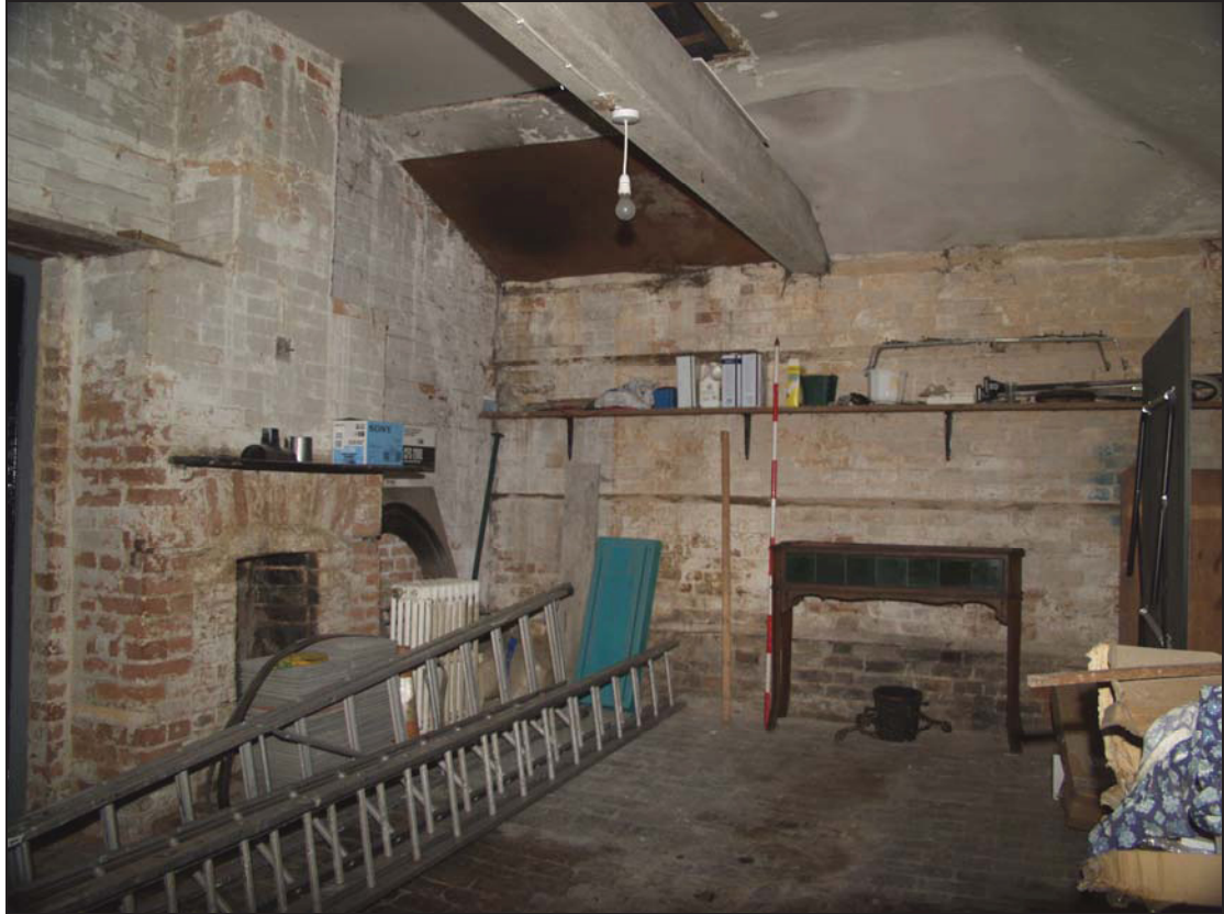
Plate 5 Interior of Building 3, taken from the north-west (22)
