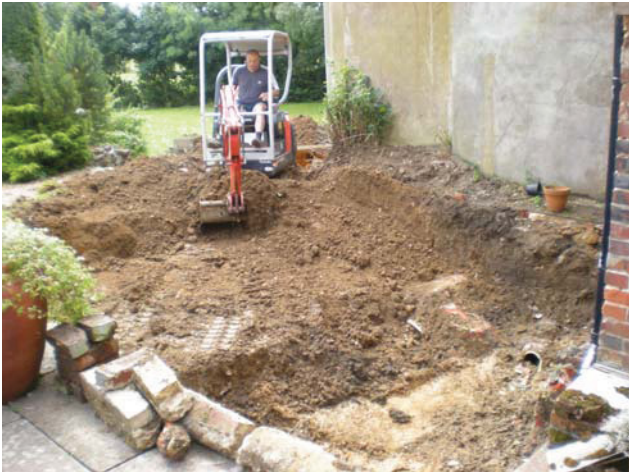
DP 3. Ground works. View S.
