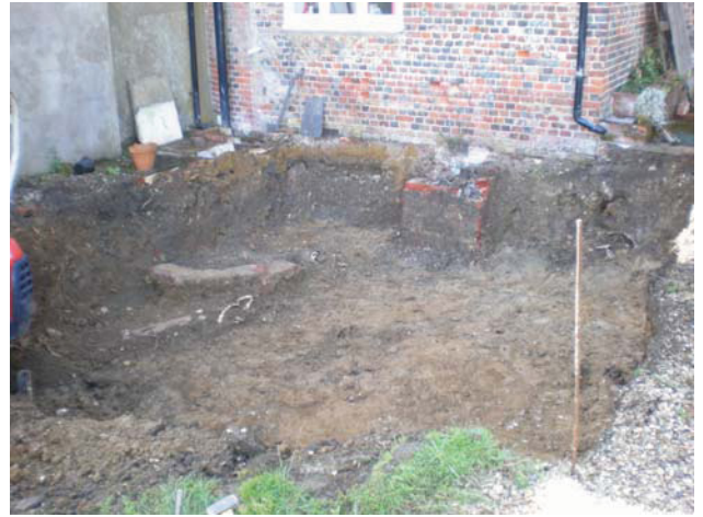
DP 4. Excavation area. View W.
