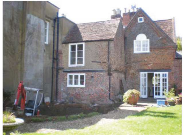
DP 2. W part of the house with excavation area. View WNW.
