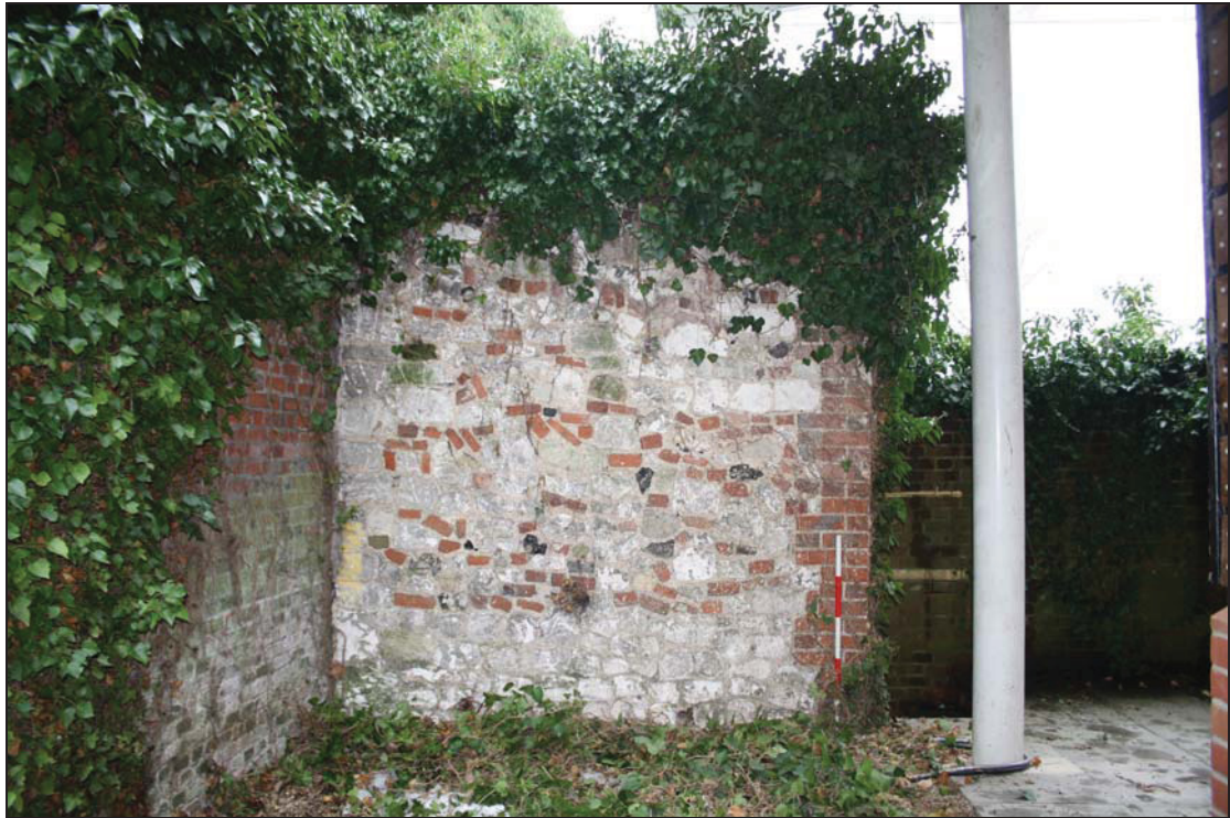
Plate 3 North face of Nib Wall 1, taken from the north (DP 07)
