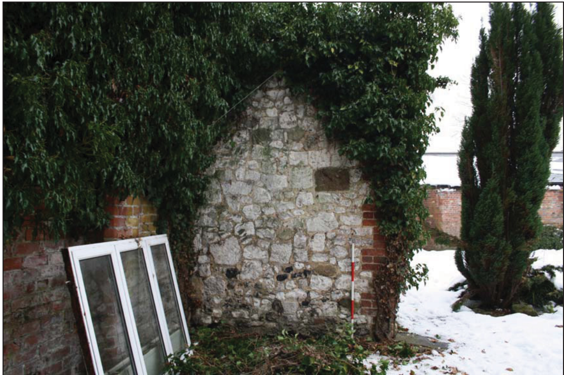
Plate 4 North face of Nib Wall 2, taken from the north (DP 11)
