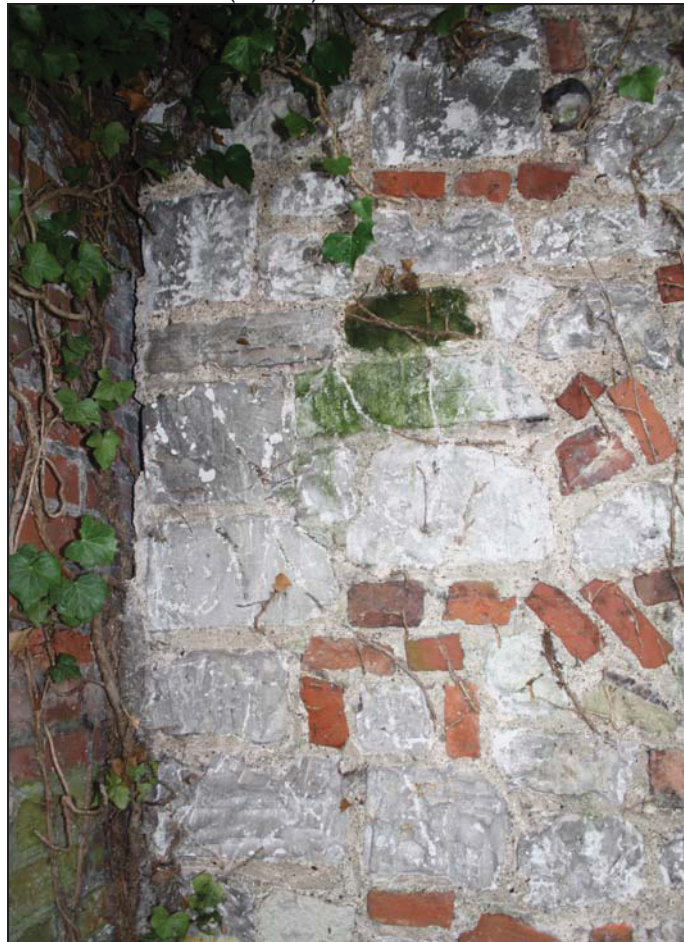
Plate 2 Detail of stone quoining on Nib Wall 1 at the junction with the retaining wall, taken from the north (DP 08)
