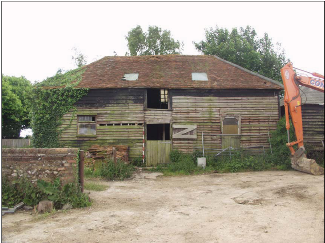
Plate 2 North façade of the barn, taken from the north (DP 15)
