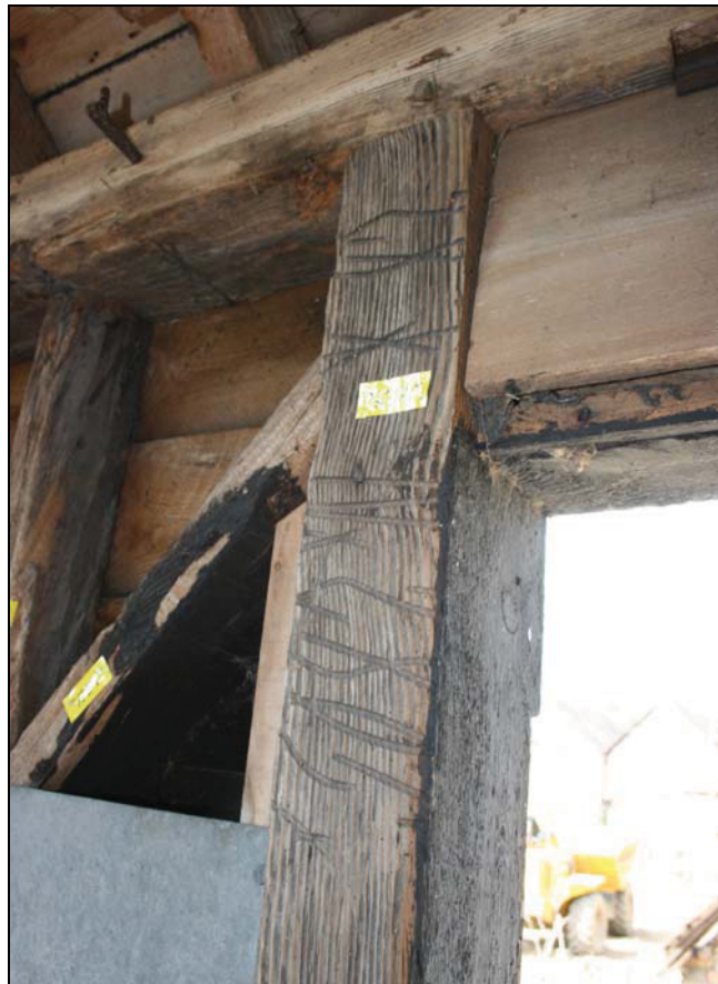
Plate 10 Baltic bracking mark on west door jamb to the granary, taken from the south (DP 33)
