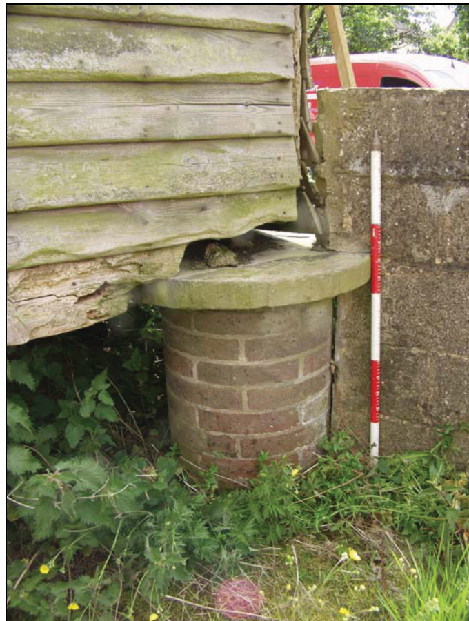
Plate 8 Brick stylobate and sandstone pad, taken from the north-east (DP 24)
