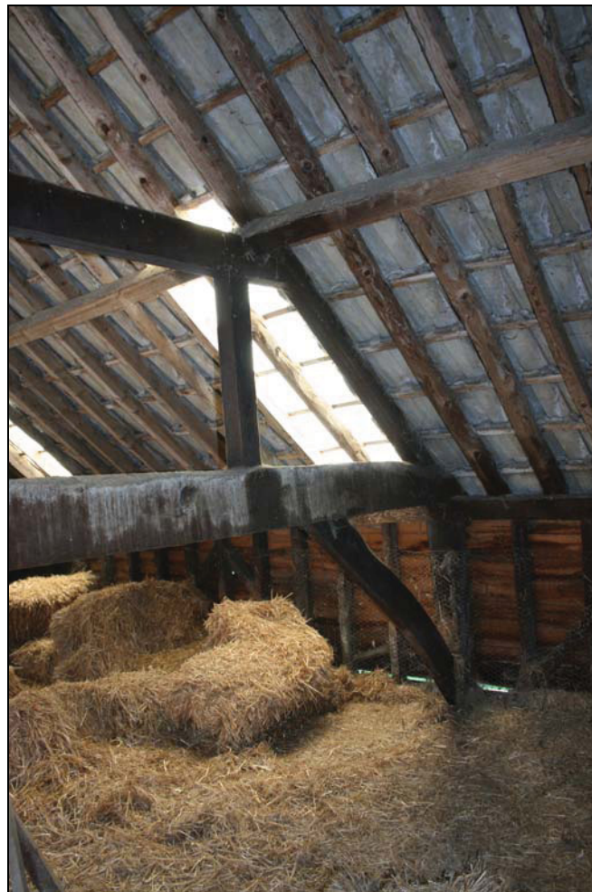
Plate 6 South side of the central truss of the barn at upper level, taken from the north-west (DP 50)
