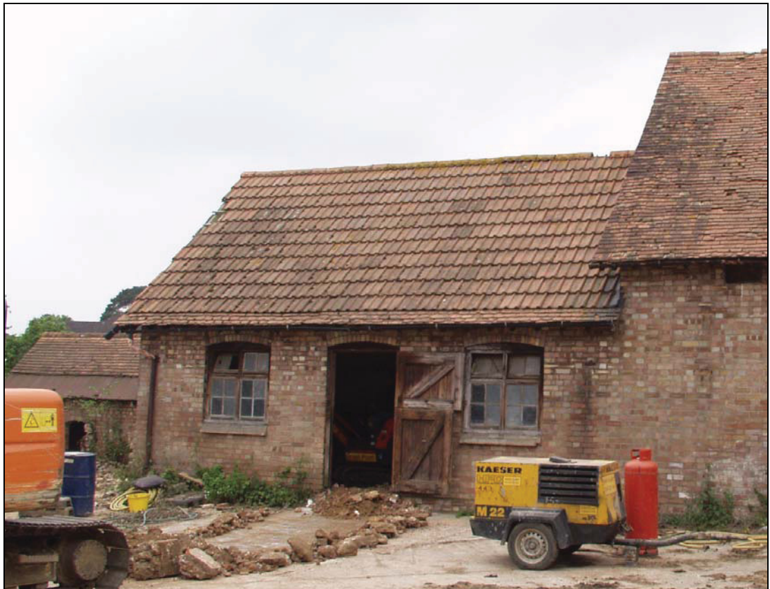
Plate 8 East elevation of Range 3 (brick barn), taken from the east (10)
