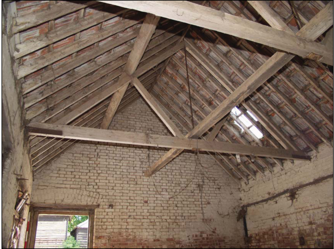
Plate 9 Roof structure of Range 3, taken from the north-east (15)
