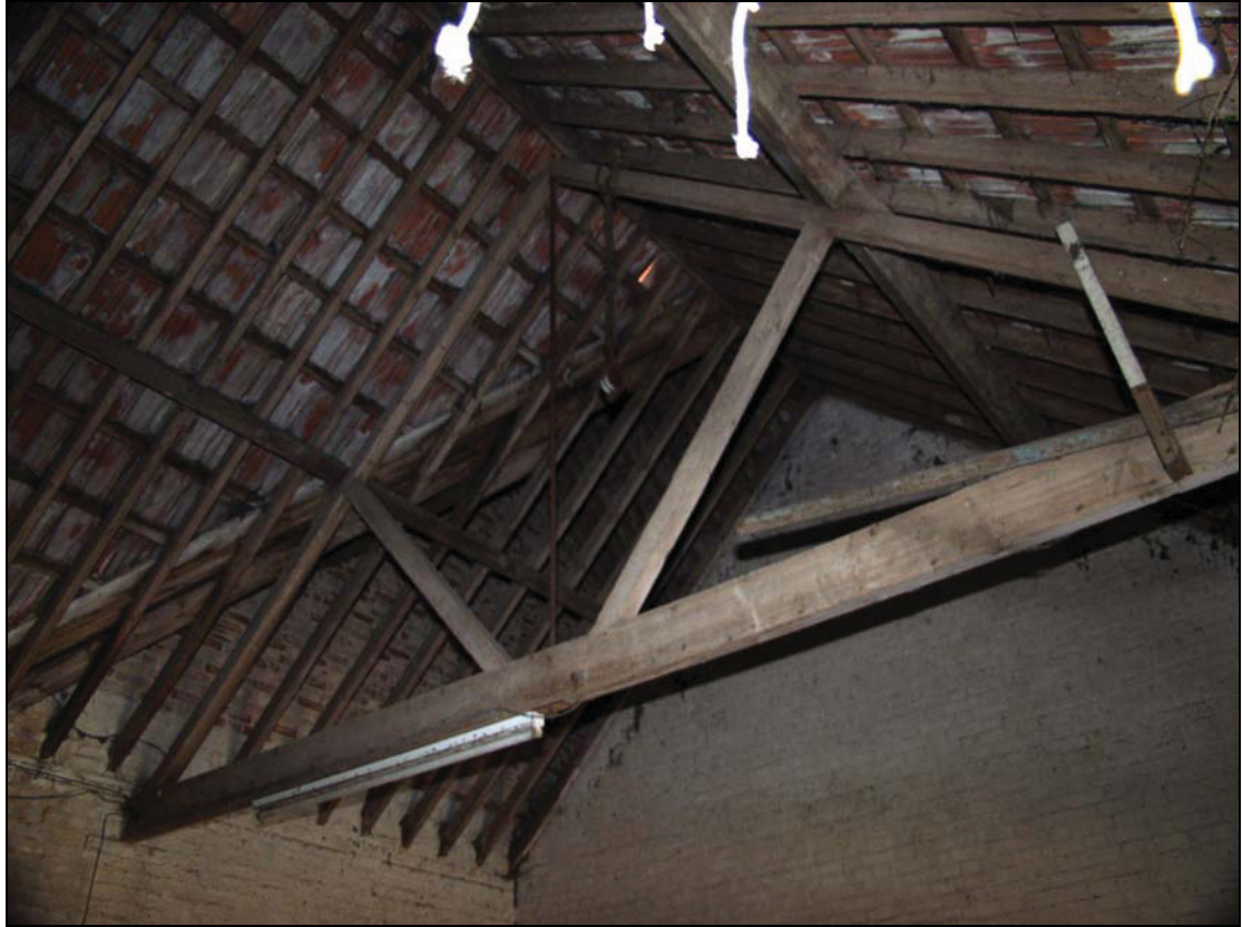
Plate 7 Roof structure of Unit 4 (Range 2), taken from the north-east (21)
