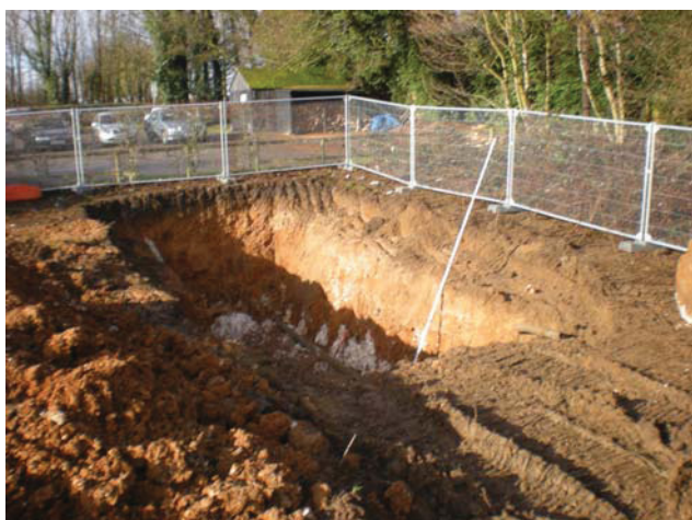
DP 3. The trench for sewage treatment plant. View NW.
