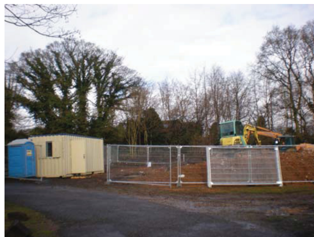
DP 2. The area of groundworks. View N.
