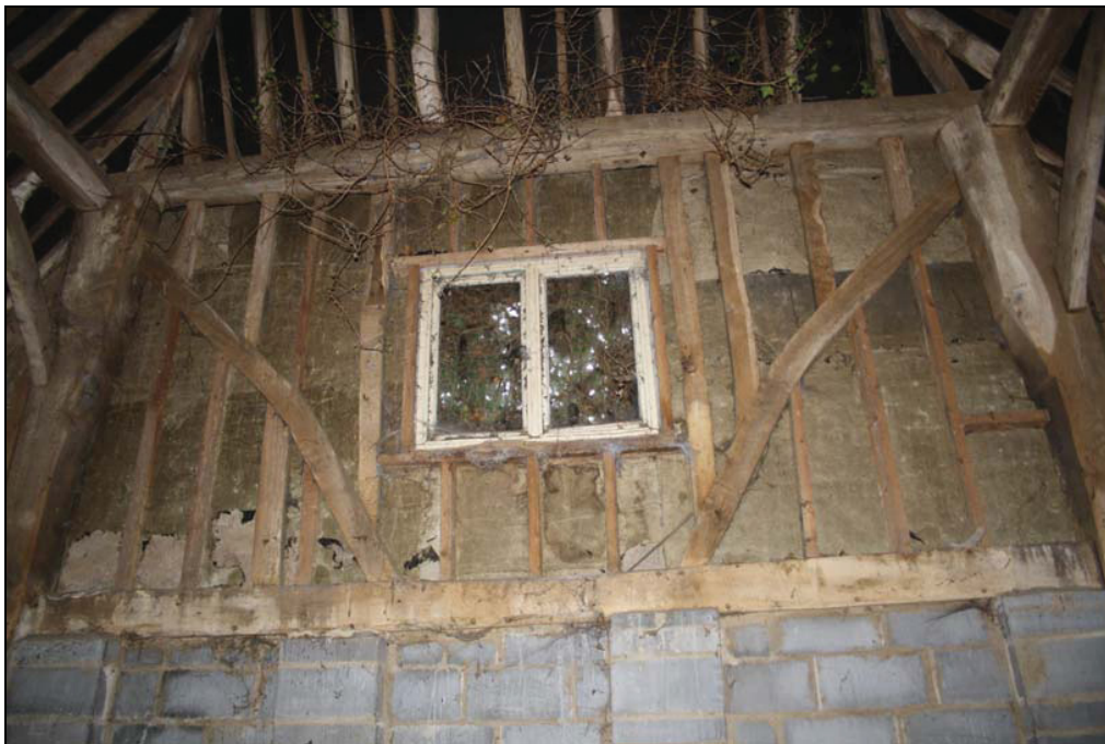
Plate 18 The barn, interior, truss 6, upper register, taken from the west (DP 42)
