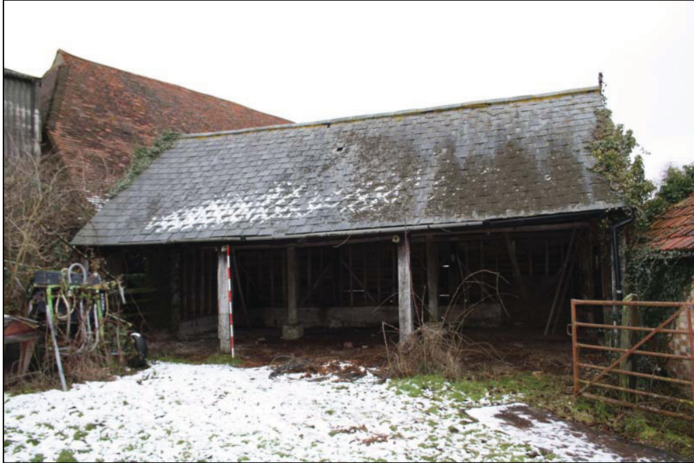
Plate 19 The cart shed, western elevation, taken from the west (DP 5)
