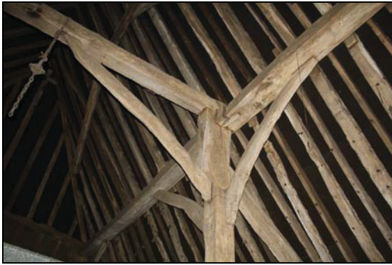
The barn, interior, truss 2, jowled arcade post and associated members, taken from the south-east
