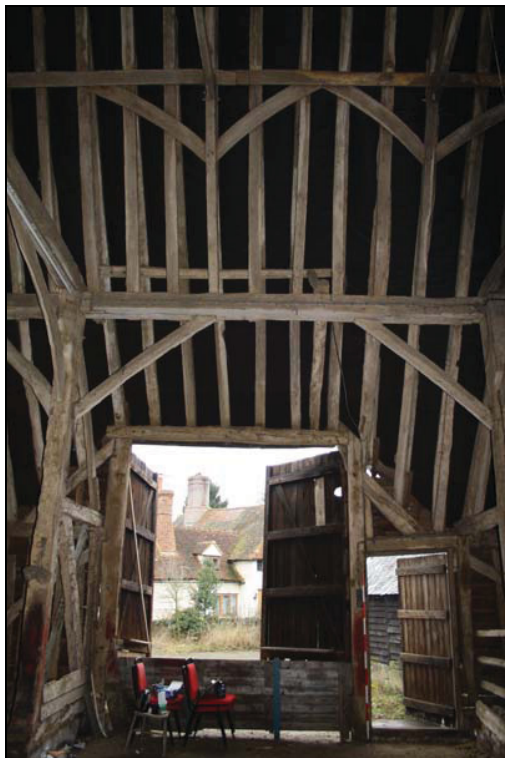
Plate 11 The barn, main entrance, bay 2, taken from the north (DP 29)
