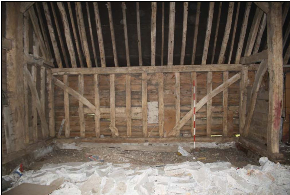
Plate 7 The barn, wall panel, bay 1, taken from the south (DP 32)
