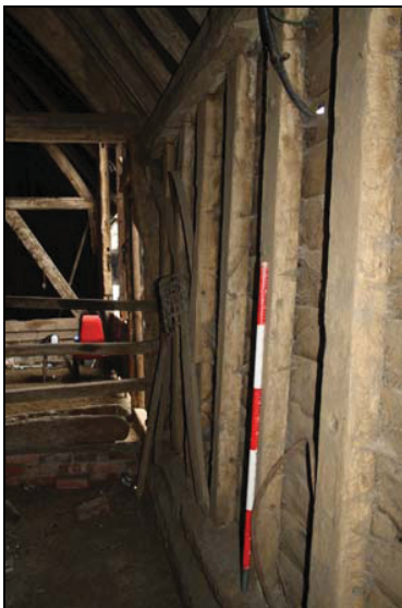
The barn, systematic wattle holes along wall panel studwork, bay 1, taken from the north-east
