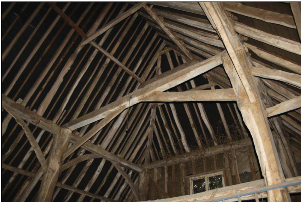
Plate 16 The barn, truss 5, taken from the south-west (DP 18)
