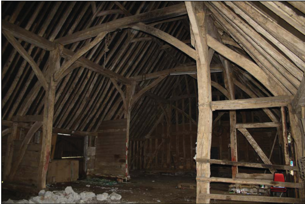
Plate 4 The barn, trusses 2 and 3, taken from the south-west (DP 37)
