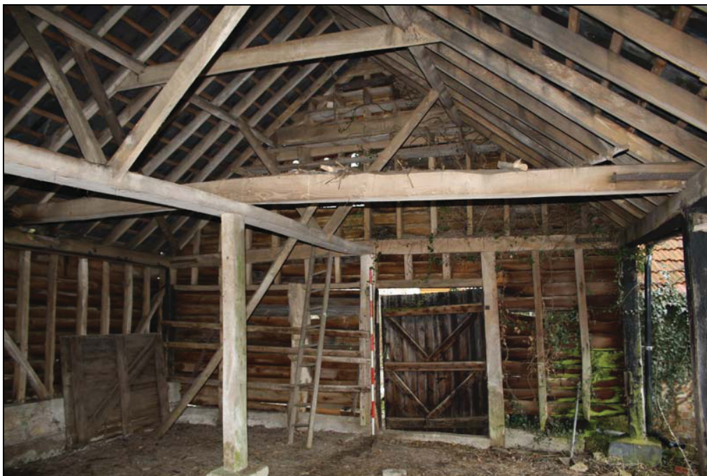
Plate 22 The cart shed, internal, southern elevation, taken from the north-west (DP 11)
