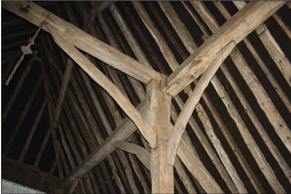
Plate 5 The barn, interior, Truss 2, jowled arcade post and associated members (DP 41)
