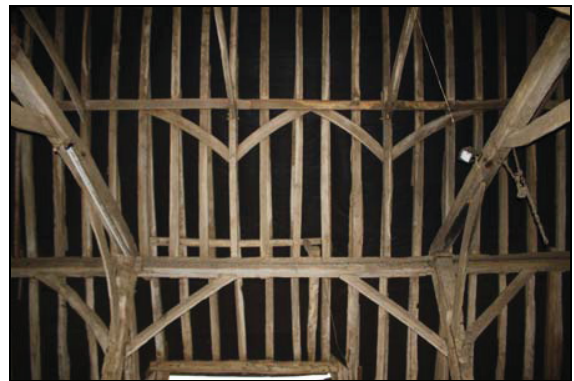
The barn, arcade plate and posts, bay 1, taken from the south-east
