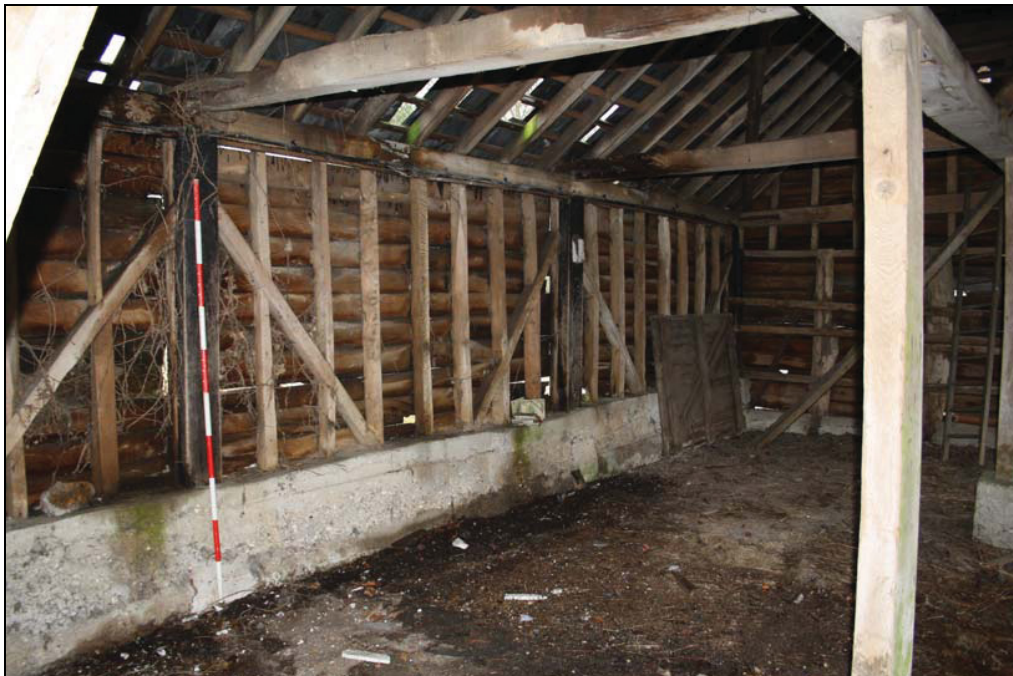
Plate 20 The cart shed, internal, eastern elevation, taken from the north-west (DP 10)
