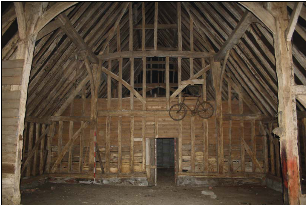
Plate 13 The barn, truss 4, taken from the west (DP 25)
