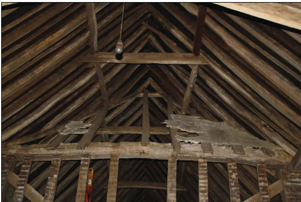
Plate 14 The barn, truss 4, original roof structure, taken from the west (DP 24)
