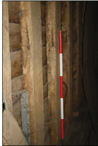
The barn, systematic wattle grooves along wall panel studwork, bay 3, taken from the south-west
