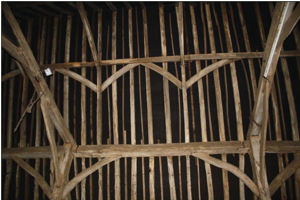
Plate 10 The barn, bay 2, roof structure, taken from the south (DP 13)
