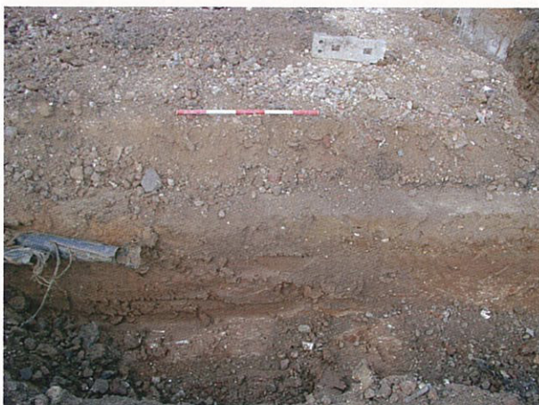
DP 17. Foundation trench, central part. Sample section. View W.
