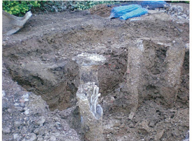
DP 20. The trench for crane base. View SW.
