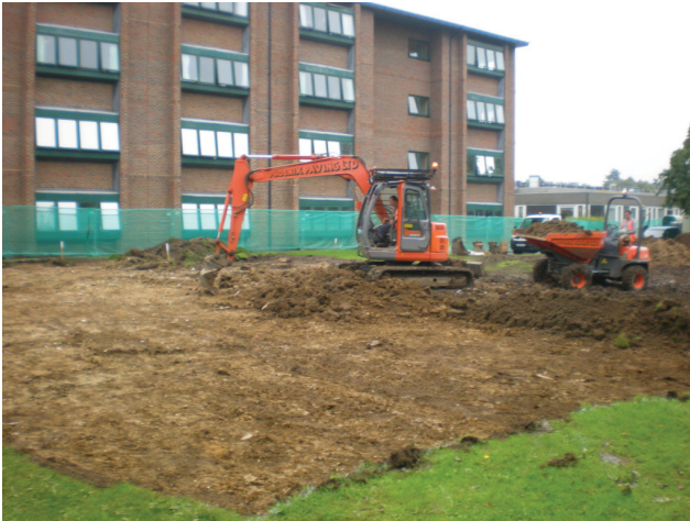
DP 3. Soil stripping. View NE.
