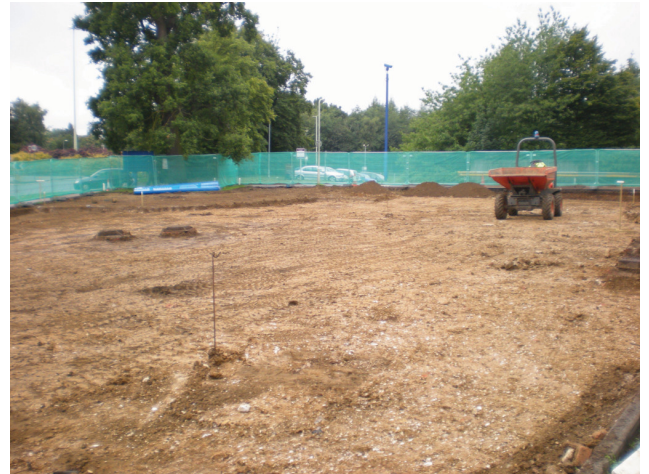
DP 4. Car park area after soil stripping. View SW.
