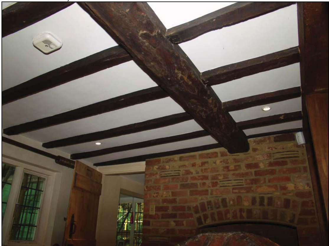
Plate 8 Exposed ceiling joists in Room 7, historic core, taken from the north-east (DP 12)
