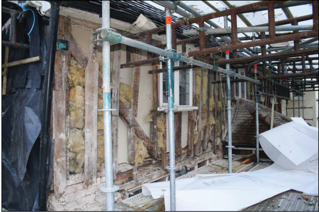
Plate 3 Timber-framing of the west bay at upper level, taken from the south-west (DP 38)
