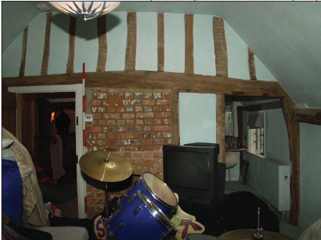
Plate 10 East side of Room 9 (historic core) adjoining the chimney bay, taken from the west (DP 28)
