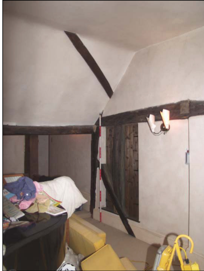
Plate 9 North-east side of Room 8 (historic core), taken from the south-west (DP 24)
