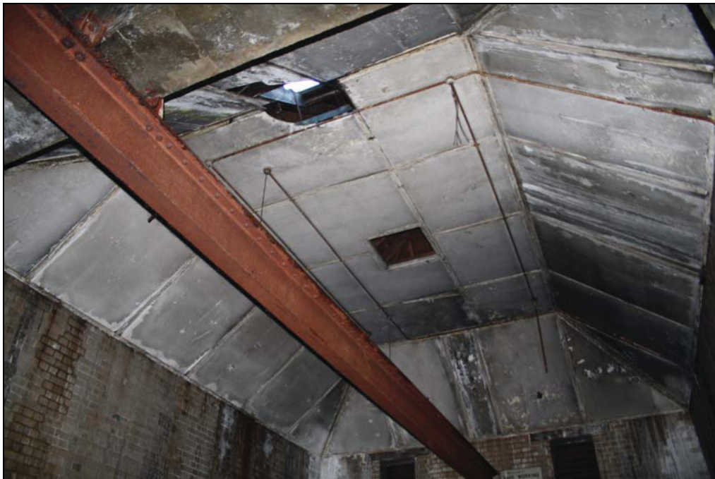
Plate 4 Engine room ceiling, taken from the north-west (DP 8)
