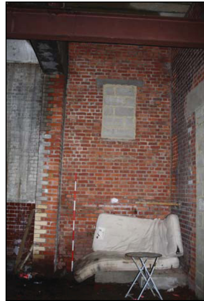
18 Extension to the engine room, taken from the east
