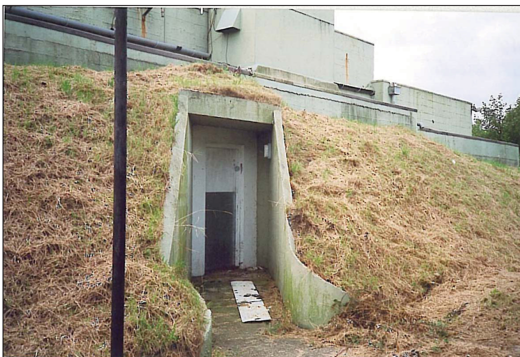
2002: As extra protection, earth was piled up all round the thick walls of the Operations Block and then grassed over. The entrance came in through the embankment.
