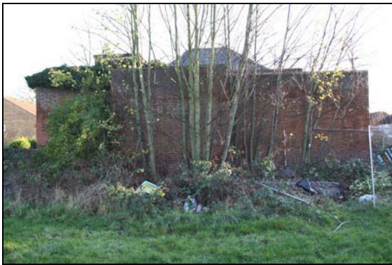
3 West elevation, taken from the west
