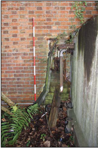
19 Fuel tank and associated pipes, taken from the west
