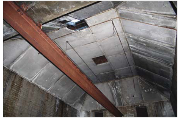
8 Engine room ceiling, taken from the north-west
