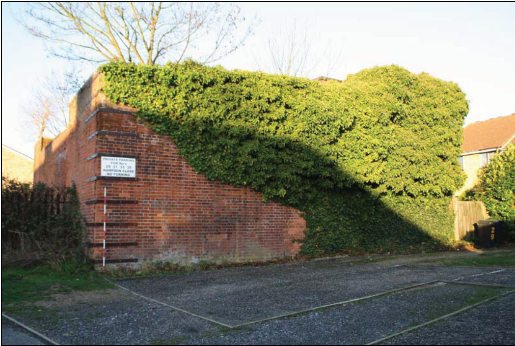
Plate 1 East elevation, taken from the south-east (DP 1)
