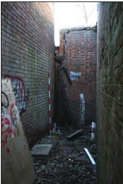
5 Area between blast wall and internal structure, taken from the north-west
