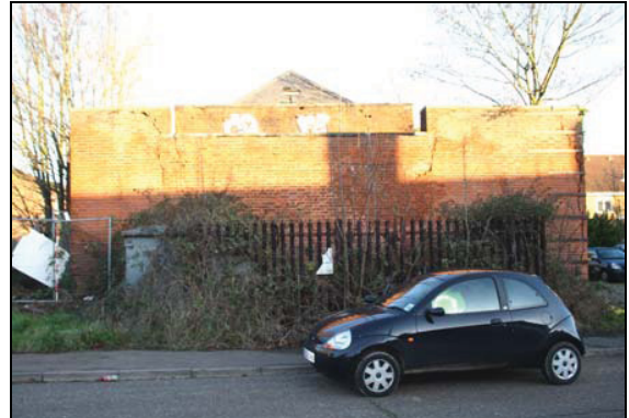
2 South elevation, taken from south
