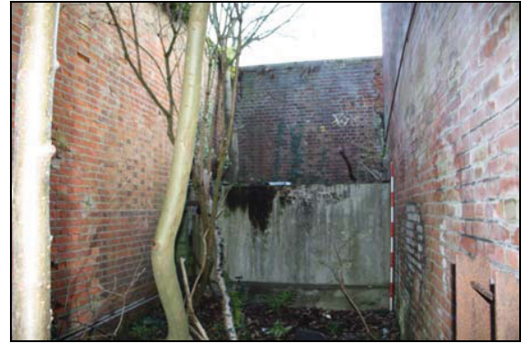
16 Fuel tank storage area, taken from the north-west
