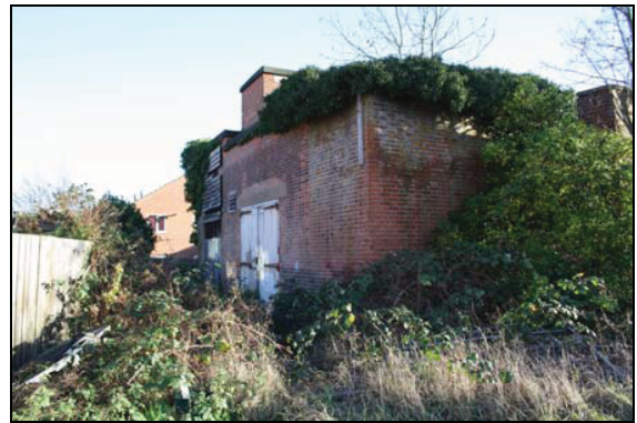
4 North elevation, taken from the north-west
