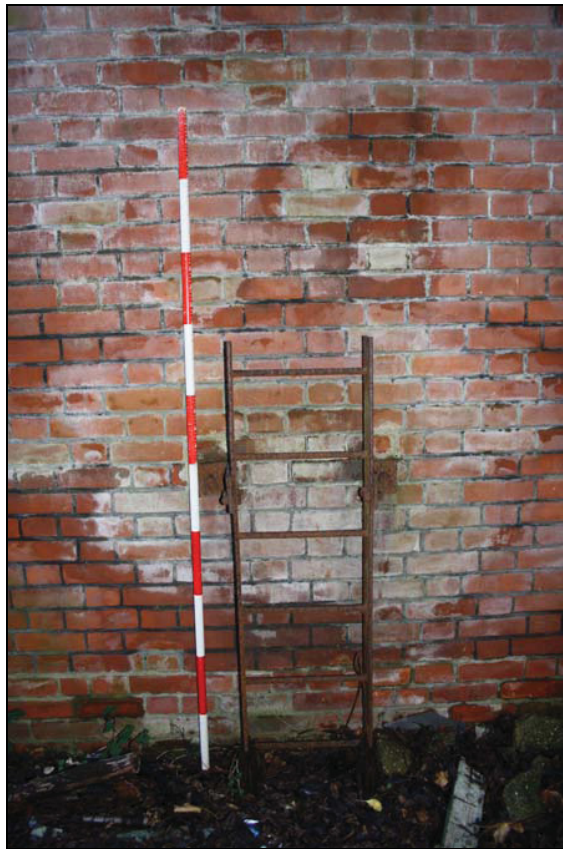
Plate 8 Metal ladder for roof access, taken from the east
