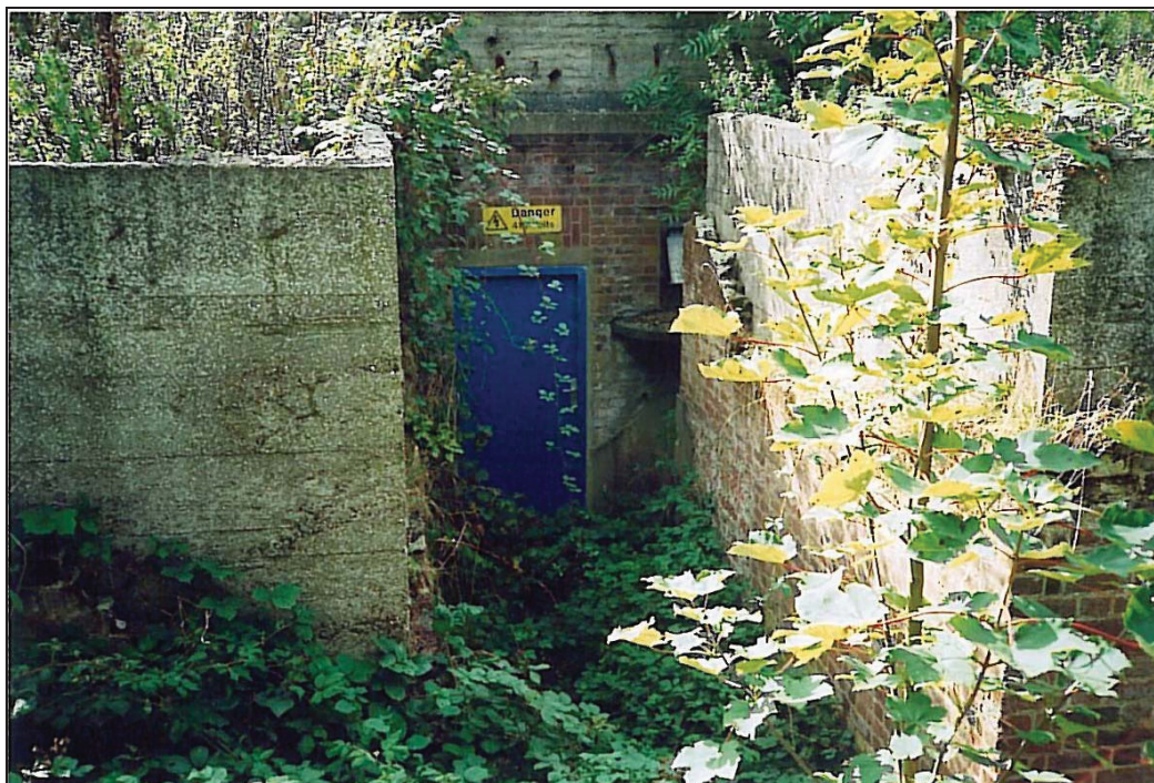
2002: The north entrance to the Sick Quarters Annex, or Decontamination Centre, protected by concrete and earth traverses.
