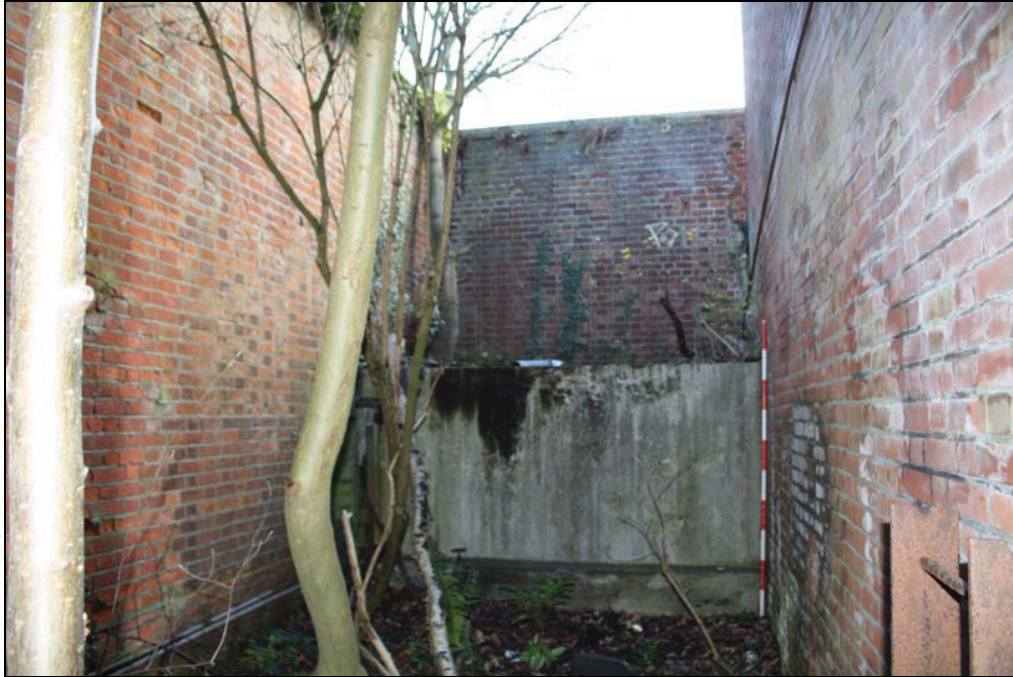
Plate 7 Fuel tank storage area, taken from the north-west (DP 16)
