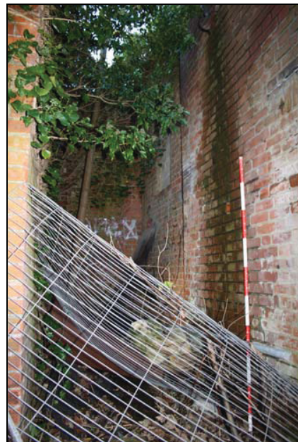
6 Area between blast wall and internal structure, taken from the south-west
