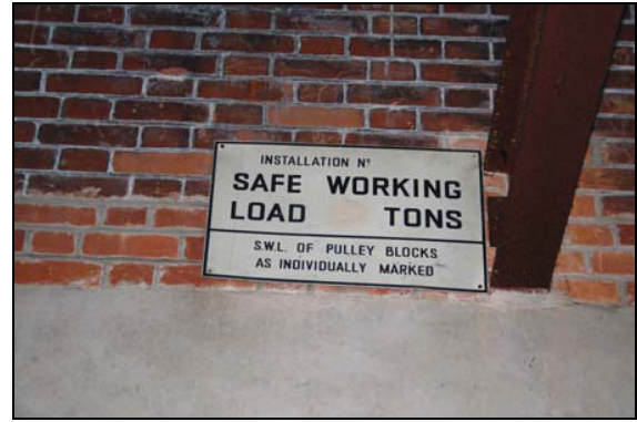
14 Safety sign for iron girder, taken from the south
