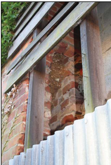
23 External blast walls showing filled cavity, taken from north-west
