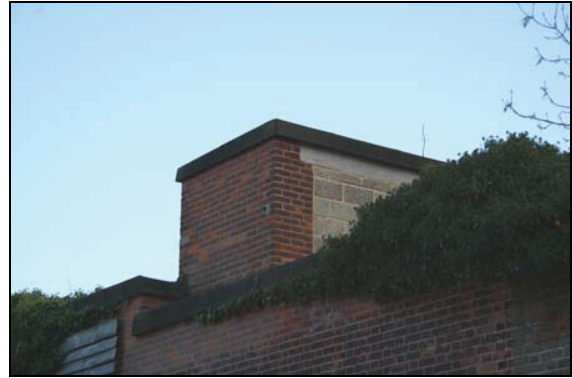
22 Brick unit on roof, taken from north-west
