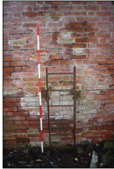
20 Metal ladder for roof access, taken from the east
