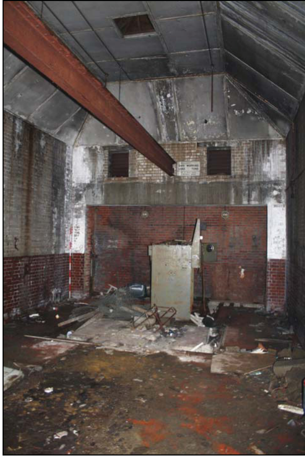
Plate 3 Engine room and machinery, taken from the north-west (DP 9)
