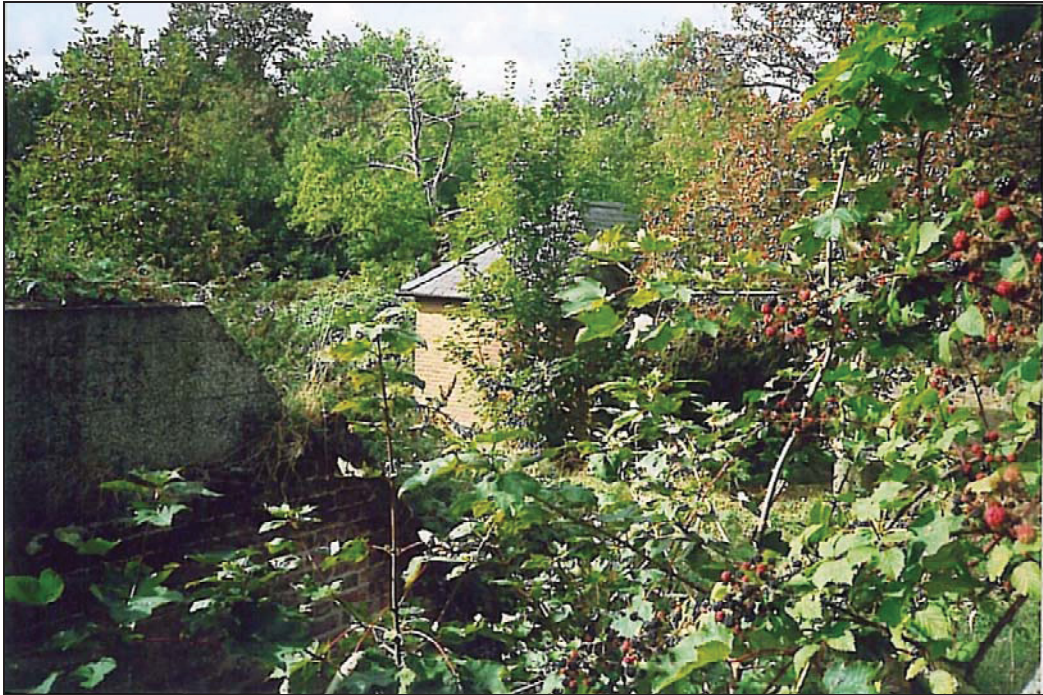
2002: The brick walls and slate roof of the Ambulance Garage through the dense thicket of the Technical Site.
