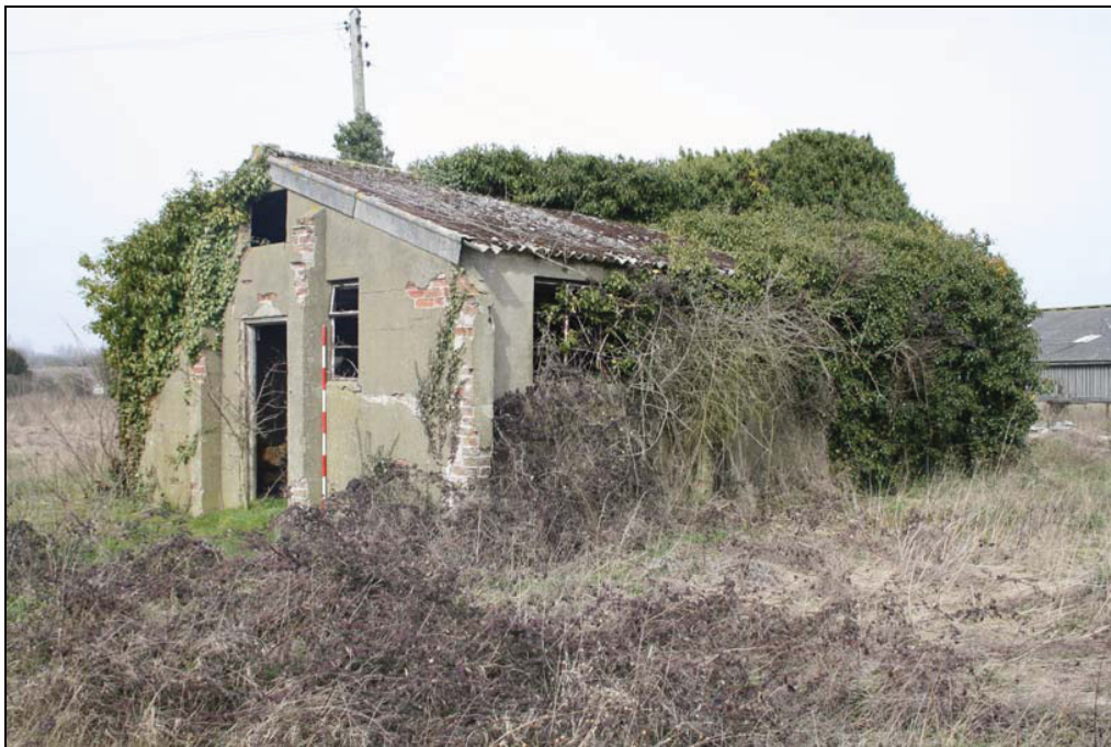
Plate 4 The airmen's latrines, taken from the south-east (DP 15)
