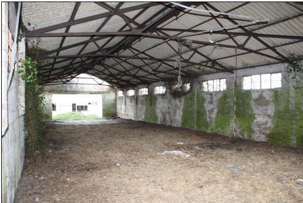
Plate 8 The gymnasium, interior, taken from the south-east (DP 39)
