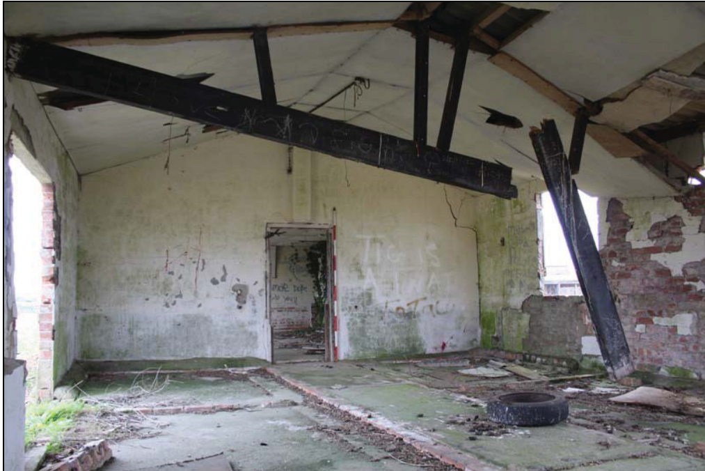
Plate 11 The meat and ration store, interior, bay 4, taken from the north-east (DP 63)
