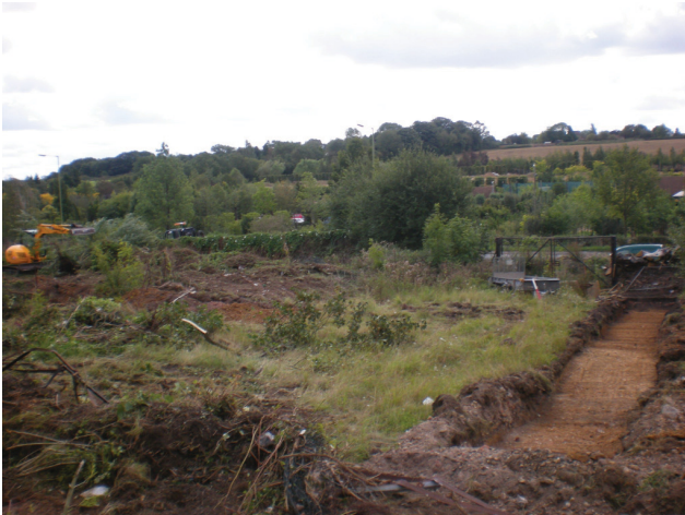
DP 3. Central part of the site with trial trenches. View SW.
