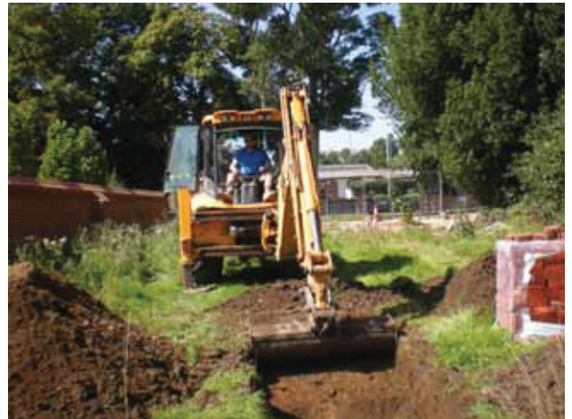
DP 2. Trial trenching in progress. View W.
