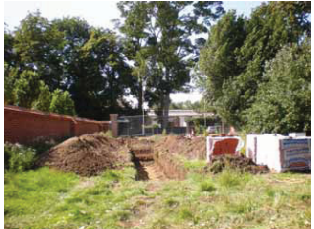
DP 4. SW part of the site with Trench 2. View W.
