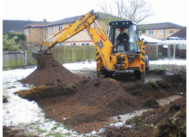
DP 2. Groundworks, Plot 1. View SW.
