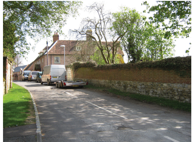
DP 2. Church Lane and Manor Farm. View E.
