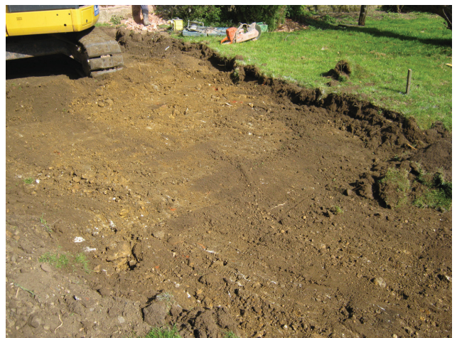
DP 6. Ground reduction for a new access road, part W. View NW.
