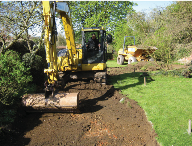
DP 3. Groundworks in progress. View W.
