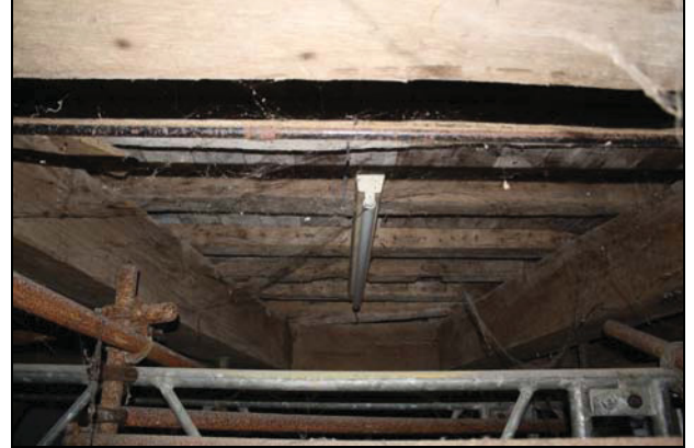
Ground floor, second bay, oak ceiling joists, taken from the south-west
