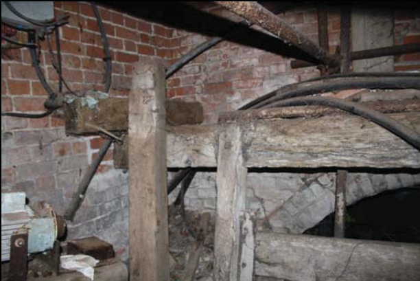
Ground floor, second bay, oak ceiling joists, taken from the north-west
