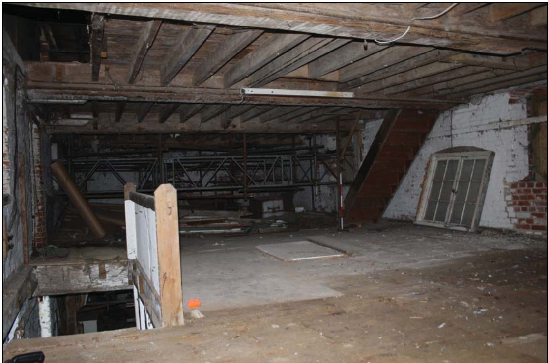
Plate 6 First floor, taken from the north-east (DP 10)
