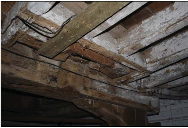
Blocked aperture possibly associated with a pulley system, taken from the east
