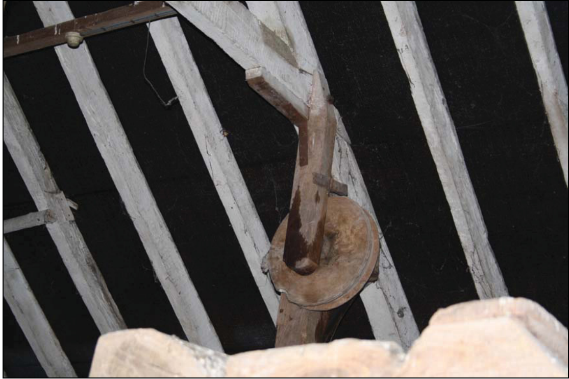
Plate 11 Pulley wheel located in roof space, taken from the east (DP 17)
