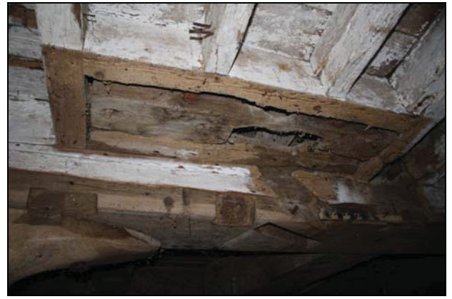
Blocked aperture possibly associated with a pulley system, taken from the east
