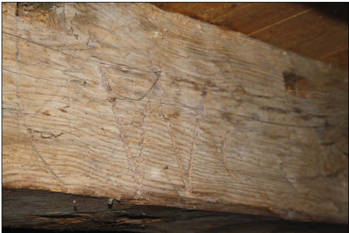
Plate 12 Detail of Baltic mark from second floor joist, taken from the north (DP 20)
