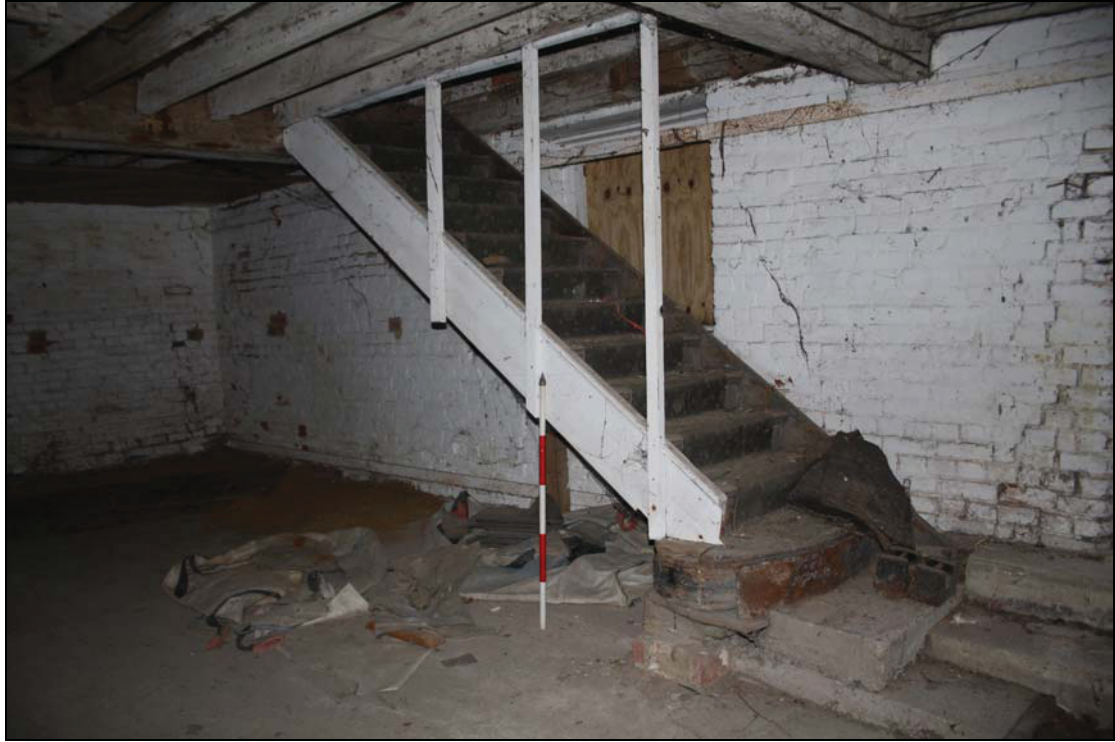
Plate 3 Ground floor reused domestic staircase, taken from the west (DP 29)
