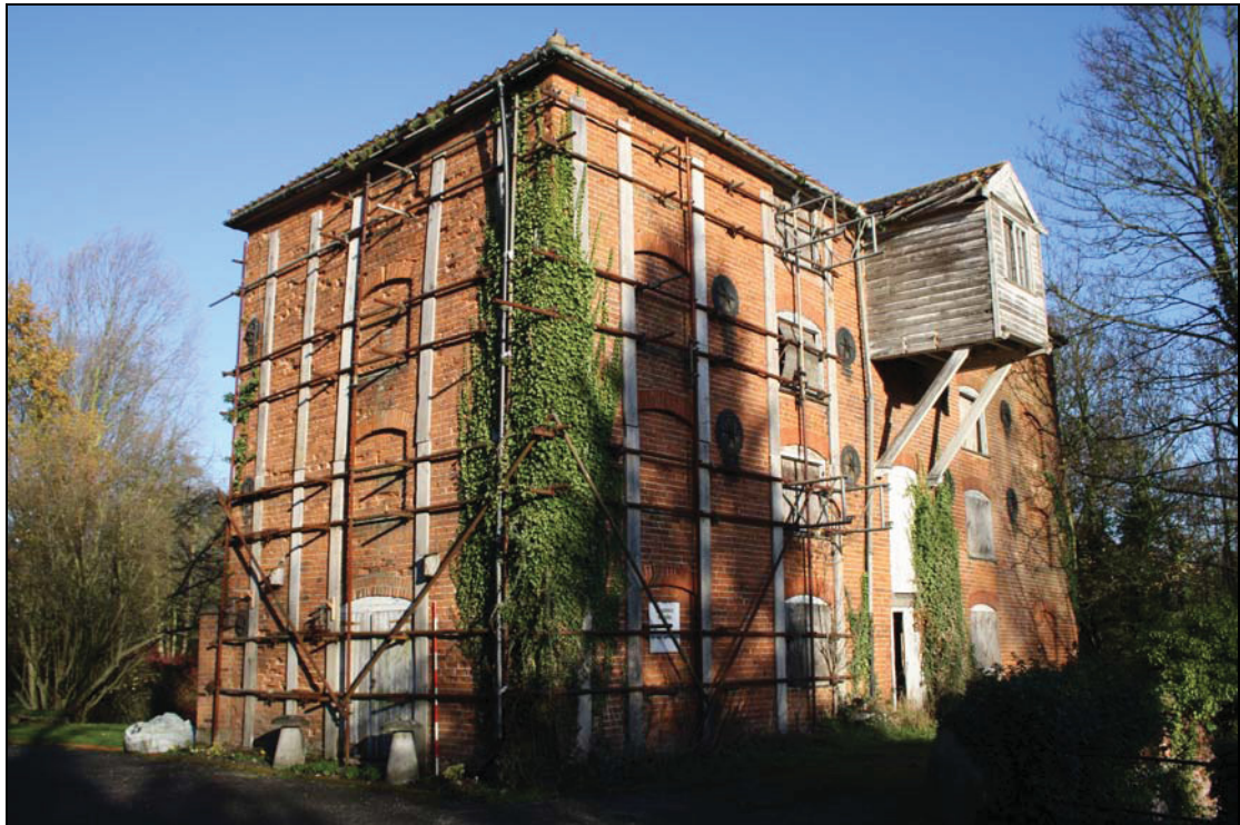
Plate 2 South-west and south-east elevations of mill, taken from the south (DP 4)
