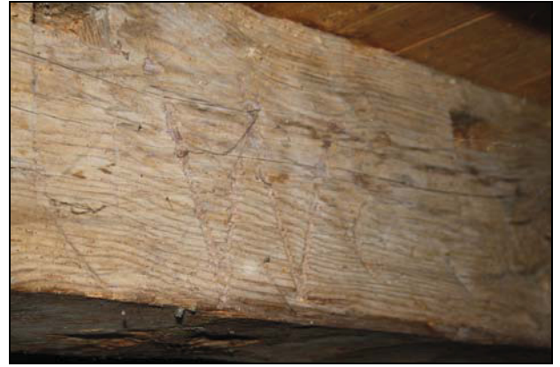
Detail of Baltic mark from second floor joist, taken from the north
