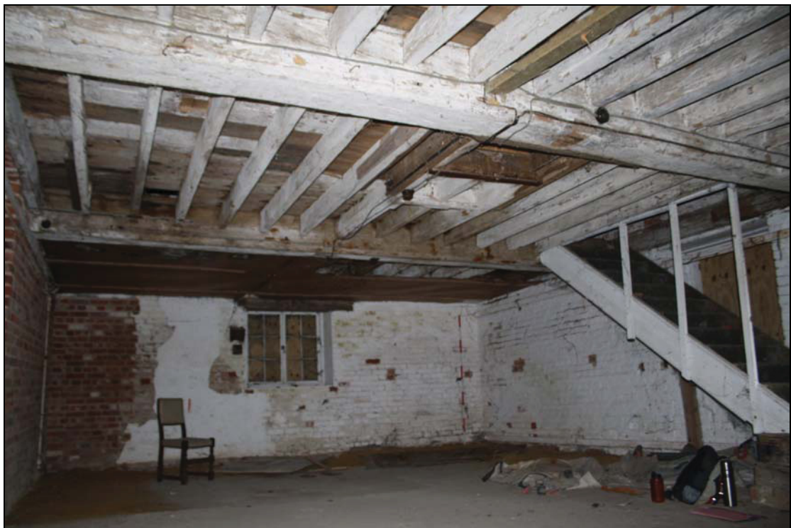
Plate 4 Ground floor, taken from the west (DP 8)
