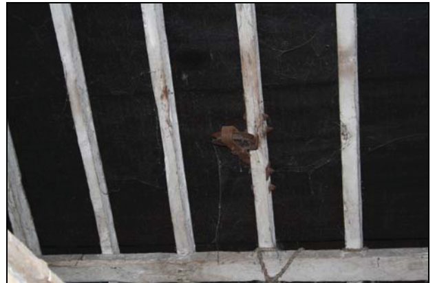
Queen post roof construction with cambered hanging joists, taken from the north-east
