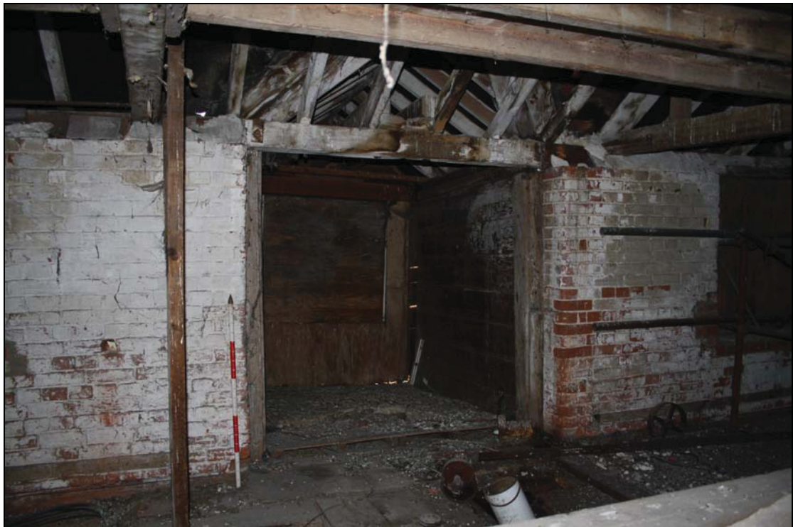
Plate 10 Hoist loft extending from south-east elevation, taken from the north-west (DP 15)
