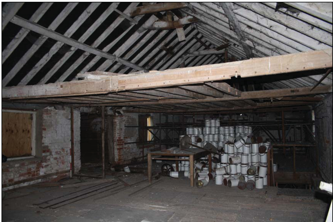
Plate 8 Third floor and roof construction, taken from the north (DP 14)
