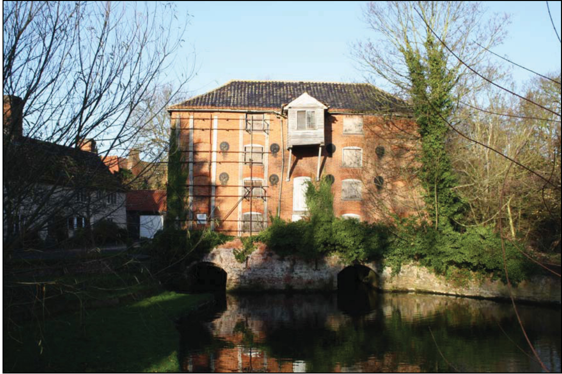
Plate 1 South-east elevation of mill, taken from the south-east (DP1)
