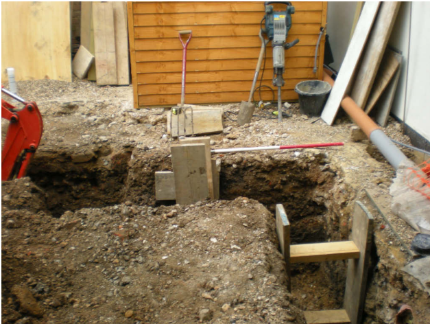
DP 3. Foundation trench in the backyard. View E.
